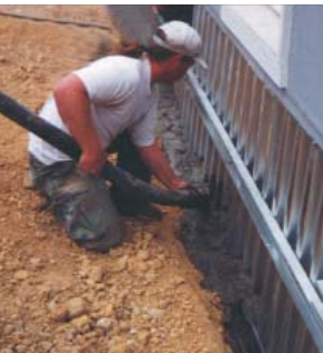
Figure 4.12 Concrete added to the trench.
