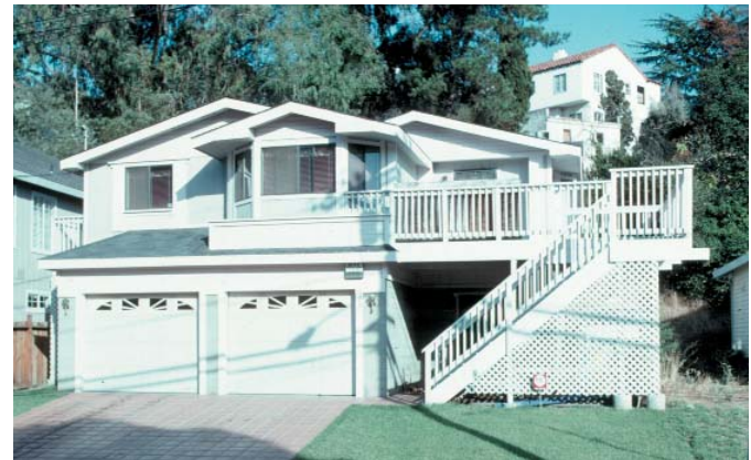
Figure 3.62 Garage/basement on upslope lot in Oakland, California.
