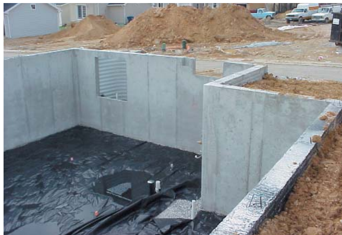
Figure 3.65 Basements are usually considered part of the living space and do not require vents for bringing in outside air.
