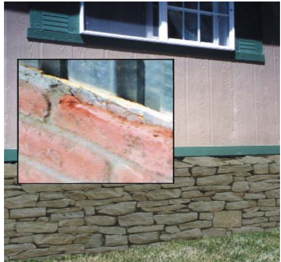
Figure 4.17 A durable base for stone cladding.
