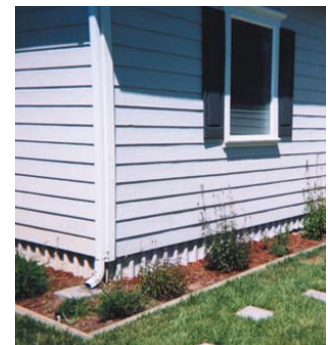
Figure 4.18 Low set, vented along the top.
