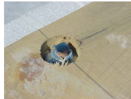
Figure 3.64 It is not recommended to core out the sill for an anchor bolt.
