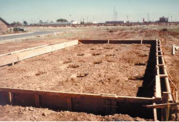
Figure 3.14 Forms ready for concrete pour.
