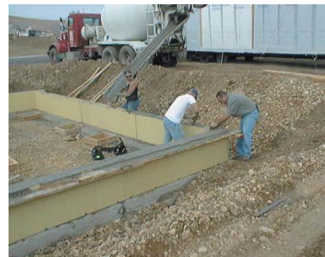
Figure 2.4 Recessing the foundation to a depth below the frost line.
