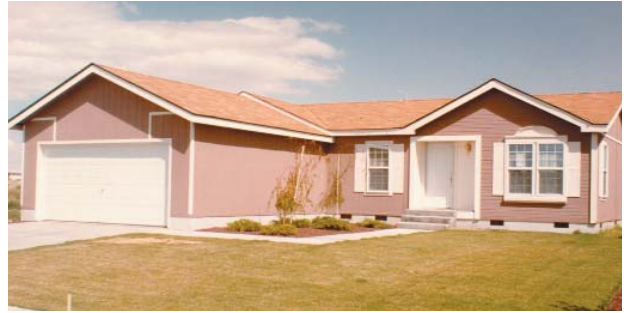
Figure 3.11 The low profile crawl space foundation system provides more of a site built appearance.
