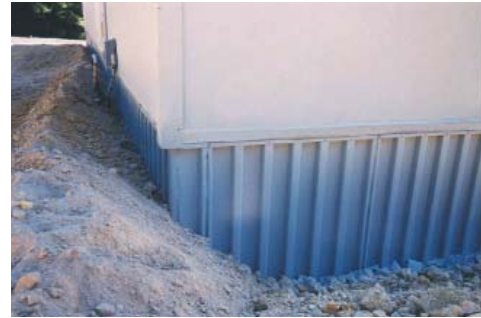
Figure 4.14 The coated panels can safely be backfilled.
