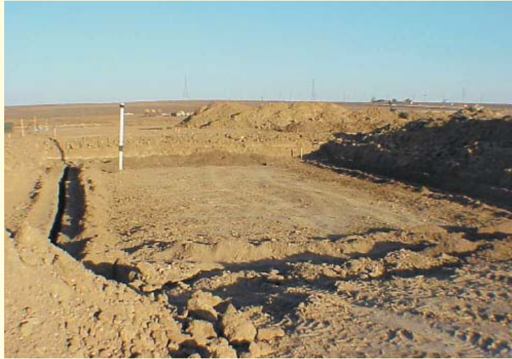
Figure 3.30 Excavation of the ground prior to setting the foundation.
