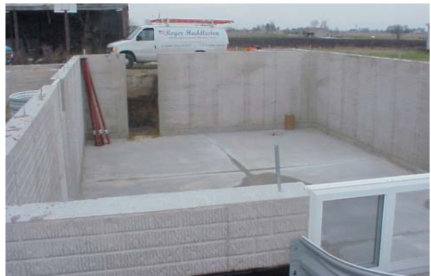
Figure 3.69 Basements are typically mostly or entirely below grade, satisfying the most stringent frost depth requirements.
