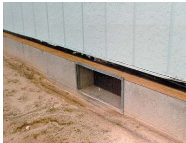
Figure 3.21 The dark horizontal area is the manufactured home floor joist, covered with the bottom board. The light wood is the foundation sill. A factory installed flashing is visible at the bottom edge of the exterior siding.
