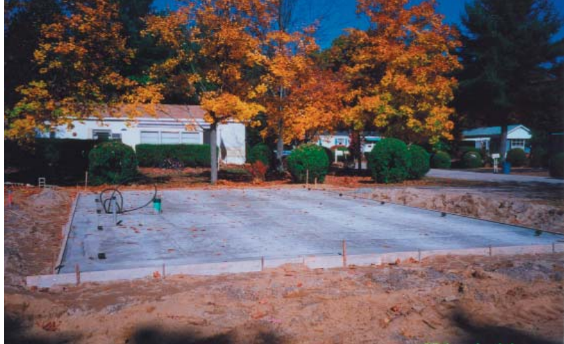
Figure 3.47 Slabs provide a monolithic structural base that if uninsulated can move with shifting soil pressures.
