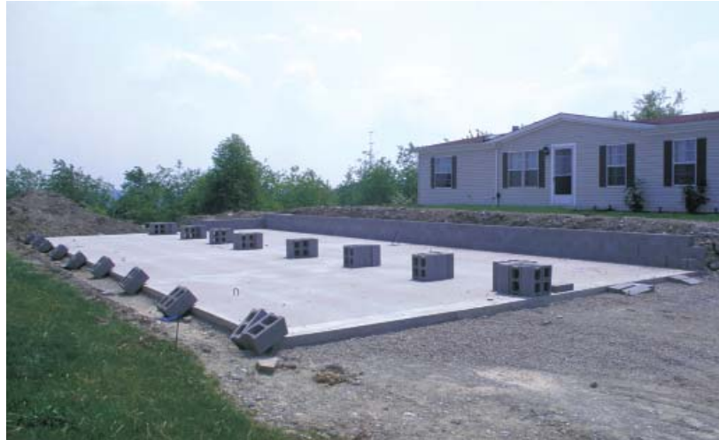
Figure 3.46 The simple design of slabs minimizes the time required for form work and provides a level base for the home.
