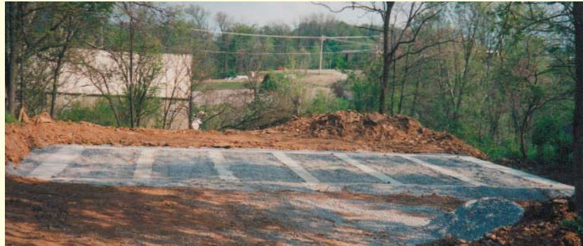
Figure 3.25 Open cells filled with crushed rock.
