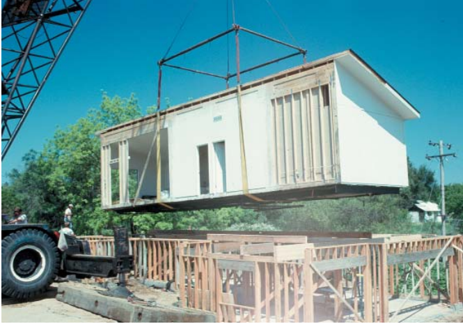
Figure 3.66 Above-ground basement with garage.
