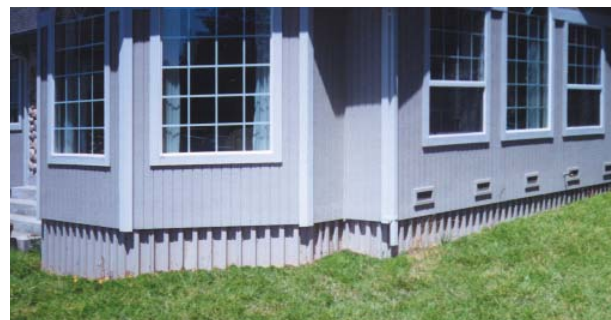
Figure 4.9 The Anchorpanel foundation simply "wraps" around difficult footprints.
