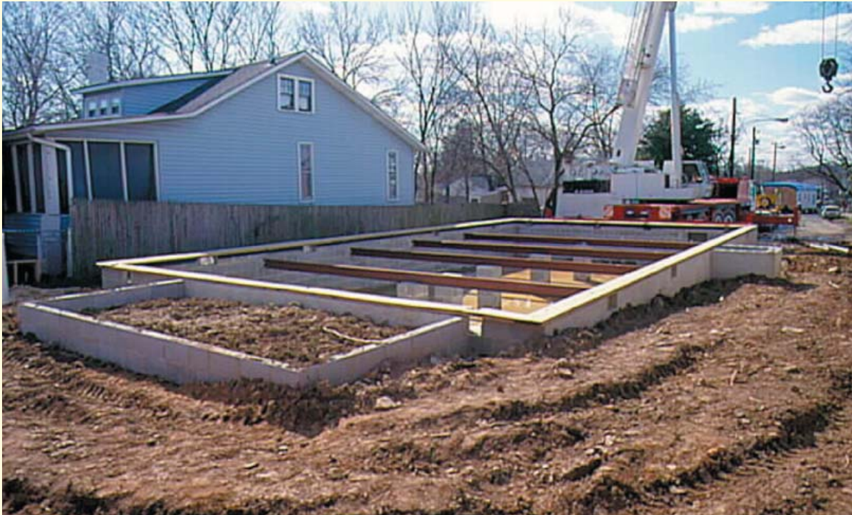
Figure 3.36 This foundation system, similar to the one used by Huddleston, is designed to carry the weight of the home at the perimeter and mating walls.
