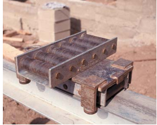
Figure 3.67 A typical roller system for conveying a home onto its foundation.
