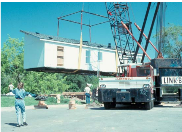
Figure 3.17 Installing a home with a crane.
