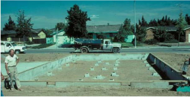
Figure 3.10 A crawl space foundation system with full perimeter support, ready for home installation.
