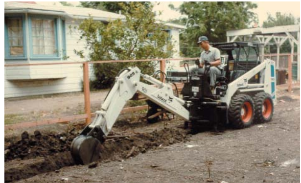
Figure 3.12 Excavating for perimeter footings with a backhoe.
