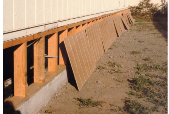
Figure 3.15 Ponywall construction method.
