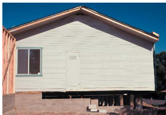
Figure 3.9 Stepped foundation.
