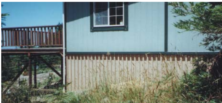
Figure 4.19 View site foundations (with decks) cost less.
