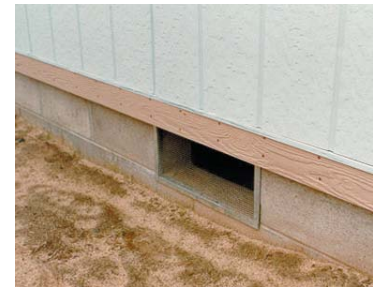
Figure 3.22 Nailing strip complete, ready for painting. When matching vertical siding is used, the joint is almost invisible from the street.
