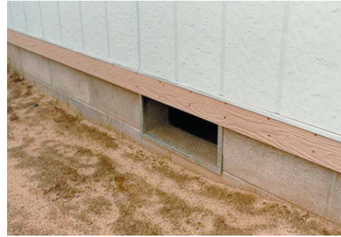
Figure 2.10 Foundation wall detail showing an air vent.
