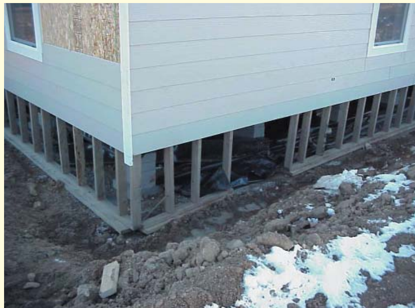
Figure 3.31 Framed stemwall sitting on concrete footer ready for siding.
