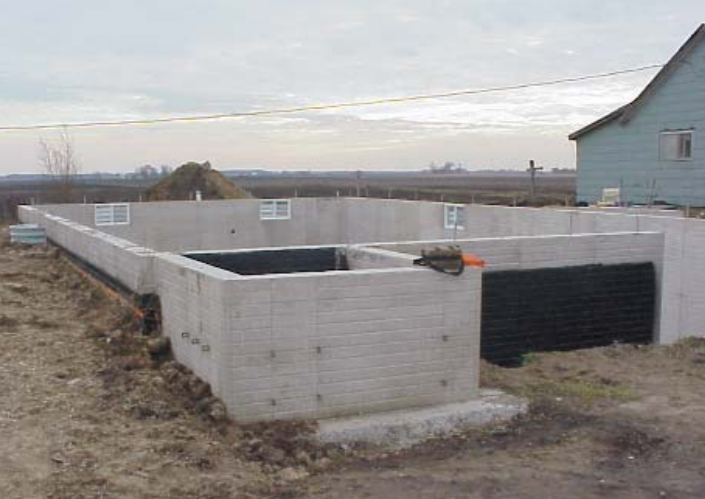
Figure 3.63 Basement showing backfill to create drainage slope.
