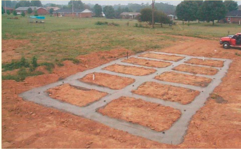
Figure 3.32 This grid-like slab can be used to support homes in a range of sizes.
