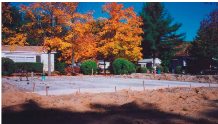
Figure 1.2 Slabs are an increasingly popular foundation system for manufactured homes, especially in the Northeast.
