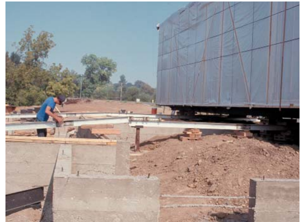
Figure 3.18 Installing a home with a roller system.
