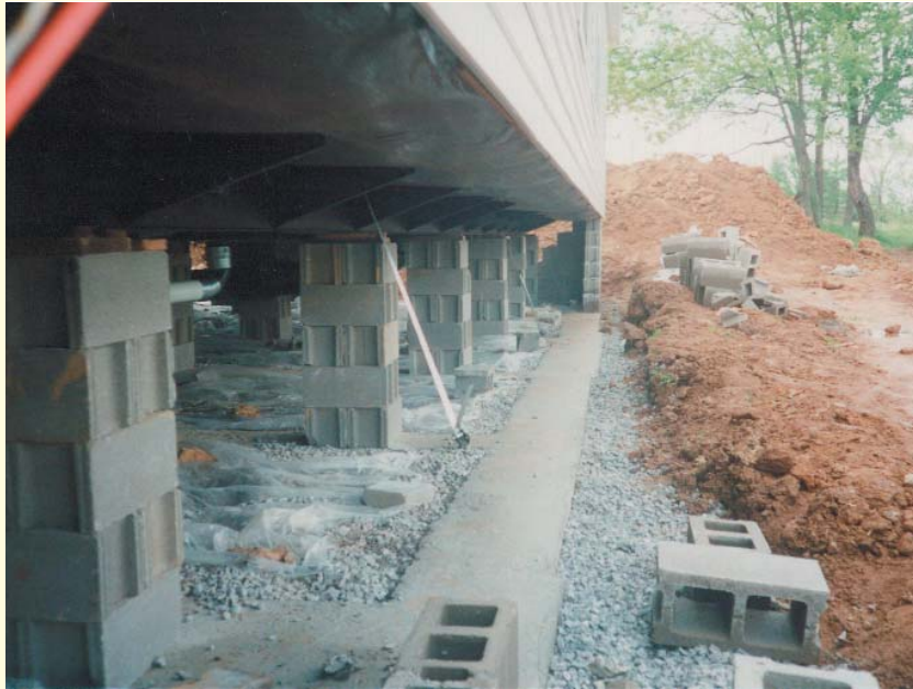
Figure 3.27 Concrete block piers support the chassis I-beams. Anchors are encased in the concrete runners.
