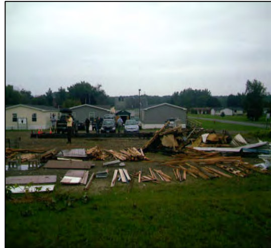
Salvaged material from the deconstruction of the two abandoned manufactured homes.
