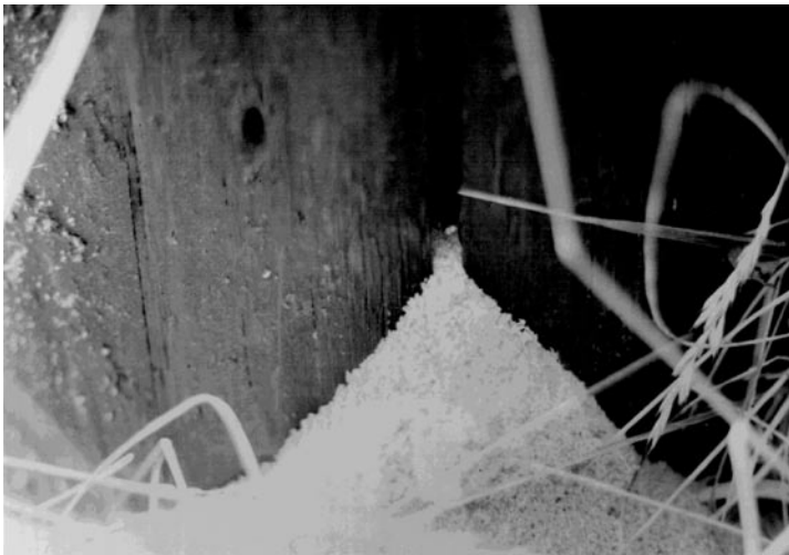
Figure 16. Carpenter ants also live in colonies, hollowing out nests in poles for shelter. A pile of sawdust at the base of the pole is a sure sign of their presence. In contrast to termites, ants have restricted waists and reproductives have shorter wings of unequal length.
