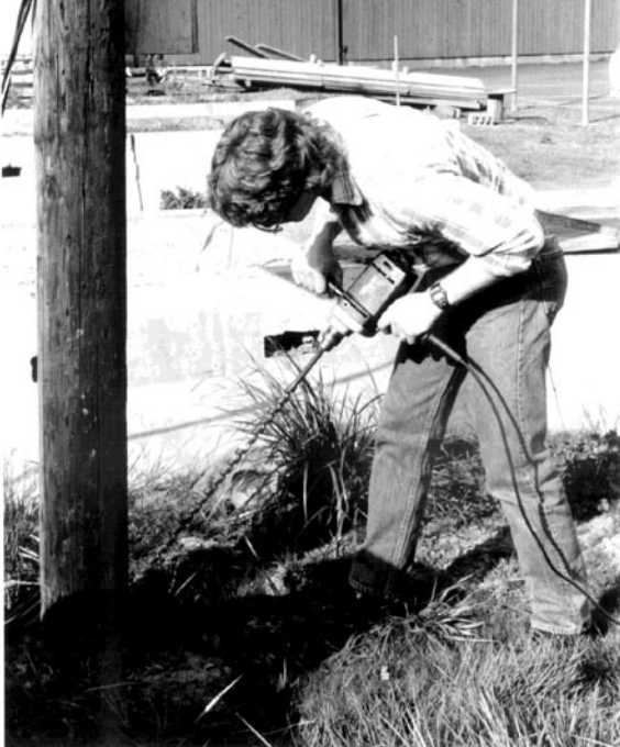
Figure 35. Fumigant application includes drilling holes at a steep angle, adding chemical, then plugging the holes.
