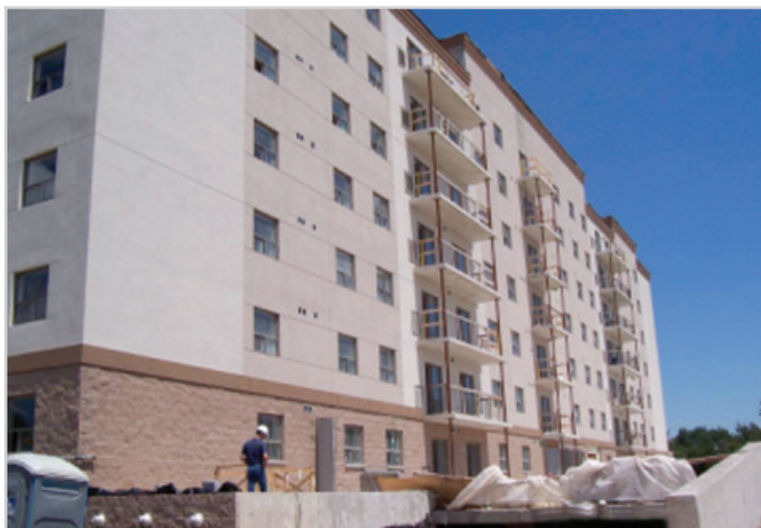
Figure 1 The building studied for the research project
