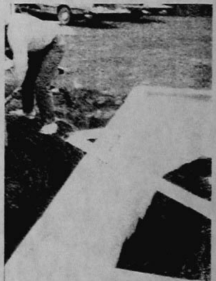
3: These polystyrene foundation forms stay in place to insulate after the monolithic slab and foundation wall is poured.
