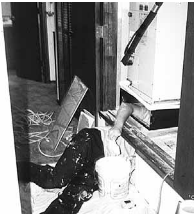
Pedestal return air: These return plenums are often very leaky and may require removing a panel to seal the leaks from inside.
