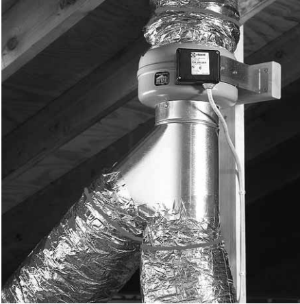
In-line fan in attic: A Y guides exhaust airflow from two bathrooms for both local exhaust and whole-building ventilation.
