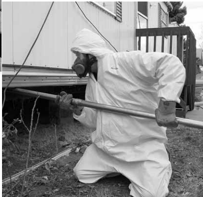
Patching a flexible belly: The technicians uses both adhesive and stitch staples to fasten a patch.
