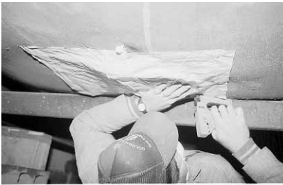
Patching a flexible belly: The technicians uses both adhesive and stitch staples to fasten a patch.
