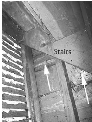
Insulating and sealing attic stair walls, doors, and stairs: Insulating and air sealing these is one way of establishing the thermal boundary.
