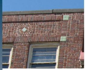
Repairs and replacement made to masonry such as that shown above should maintain the appearance of the historic patterns of bricklaying and profile, color, and texture of joinery.
