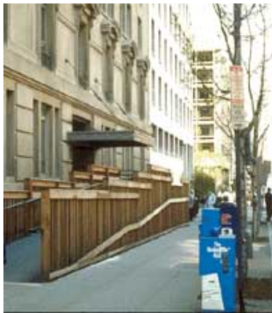
The ramp's scale and materials are inconsistent with the historic character of the building. Photo: NPS files.
