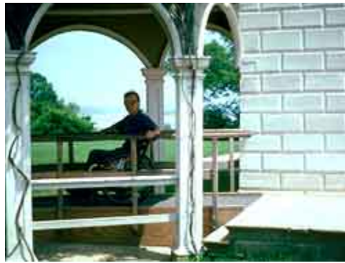
The significant building site is now accessible to people with disabilities (note steps in front of ramp). Photo: NPS files.
