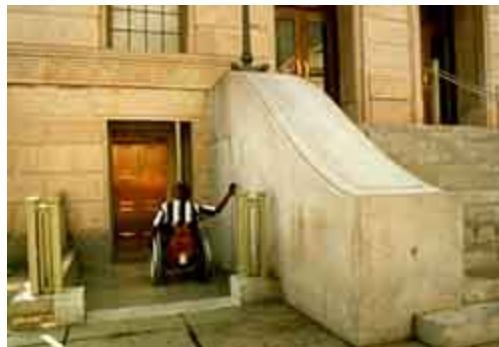
A new elevator entrance was provided next to the stairs to provide universal access to the services inside. Photo: Courtesy, GSA.
