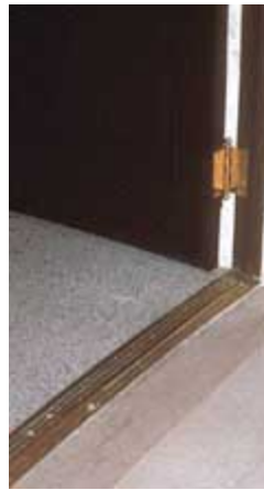
The historic threshold was made accessible with a 1/2" wood bevel. Photo: NPS files.
