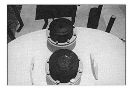
Figure 17 This 12,000-gal aboveground storage tank is constructed with integral secondary containment. The tank has two emergency vents.
