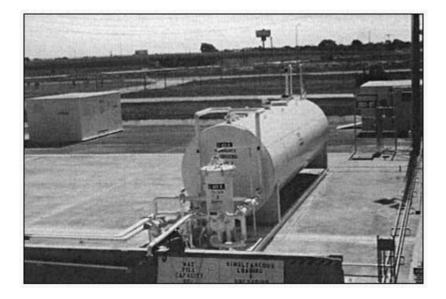
Figure 2 An uninsulated aboveground storage tank may be acceptable to the jurisdiction if it is located far enough from potential exposures.
