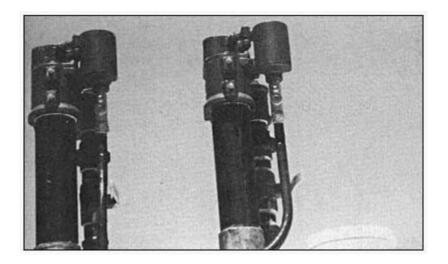
Figure 24 This tank is equipped with two listed submersible pumps used for delivering fuel oil to generator sets. These pumps have a maximum discharge pressure of 50 psig, as required by UL 79.
