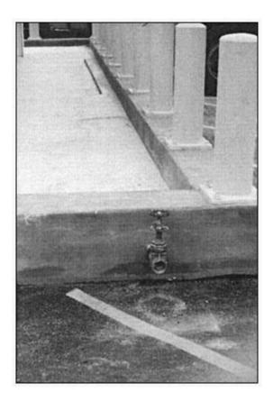
Figure 12 A method of removing water from a secondary containment is required. In this case a valve is used. Note that valve is not locked closed.
