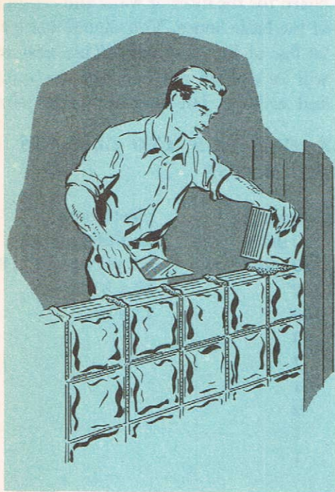
Fig. 1. When glass blocks are to be used for exterior walls, they must always be set up in mortar.
