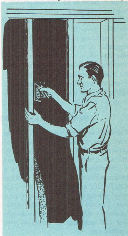
Fig. 4. Applying insulation with a special stapling machine is a great time saver.
