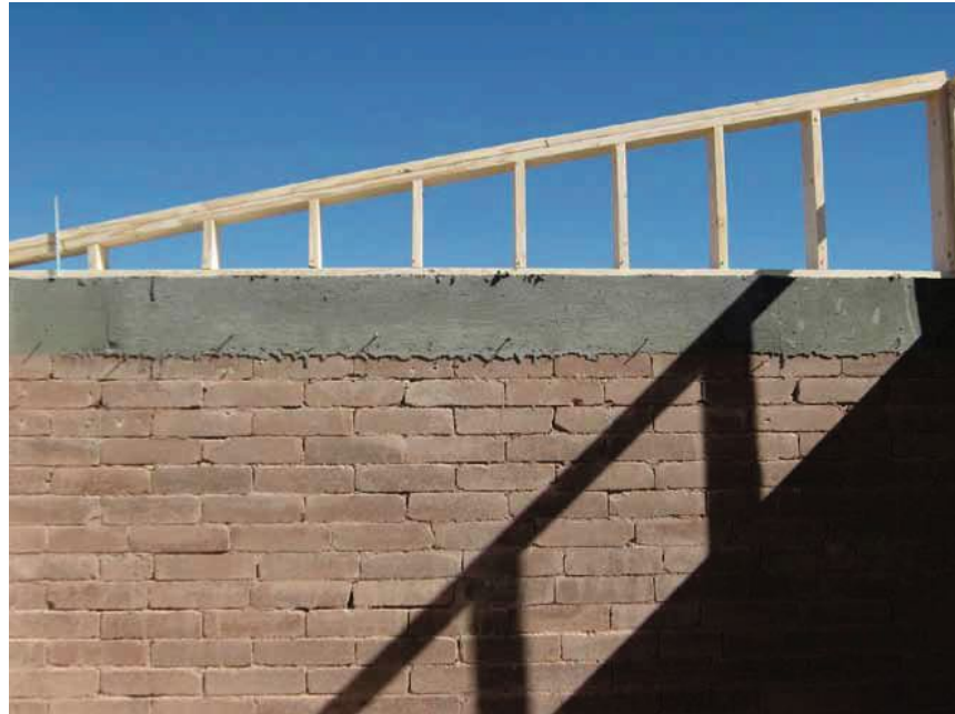
Figure 12. Finished Bond Beam With Shed Roof Framing
