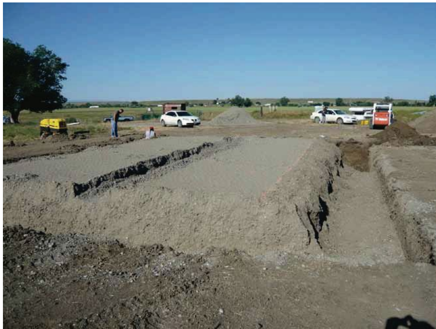
Figure 9. Over-Excavated, Compacted, Filled, and Shaped Subfoundation
