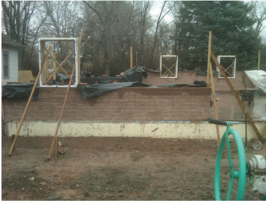
Figure 10. Window Bucks Installed
