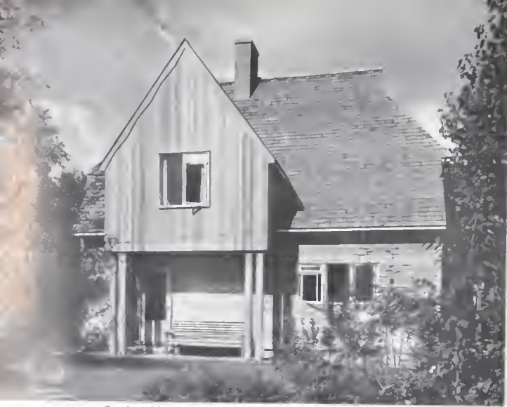
Garden side of Coronation House showing verandah
