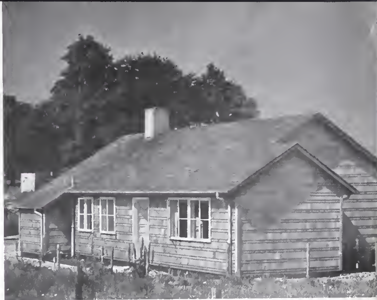
Entrance front of a modified 10A at Inverness.
