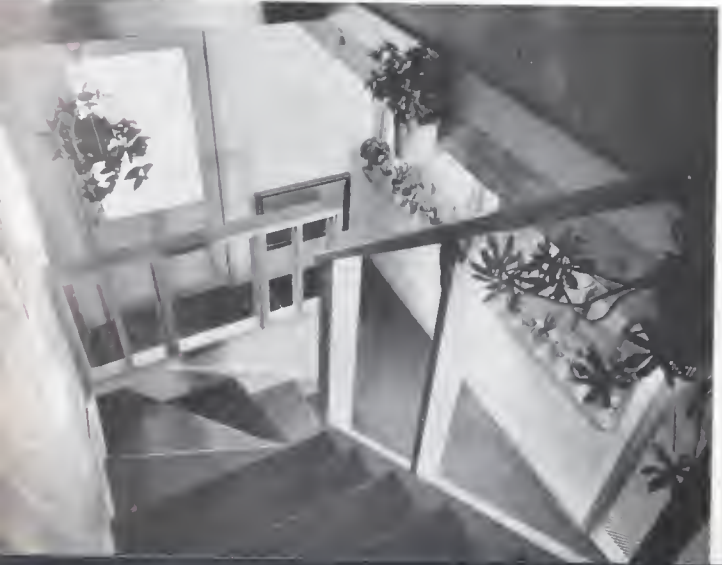
View of hall showing cork covered staircase
