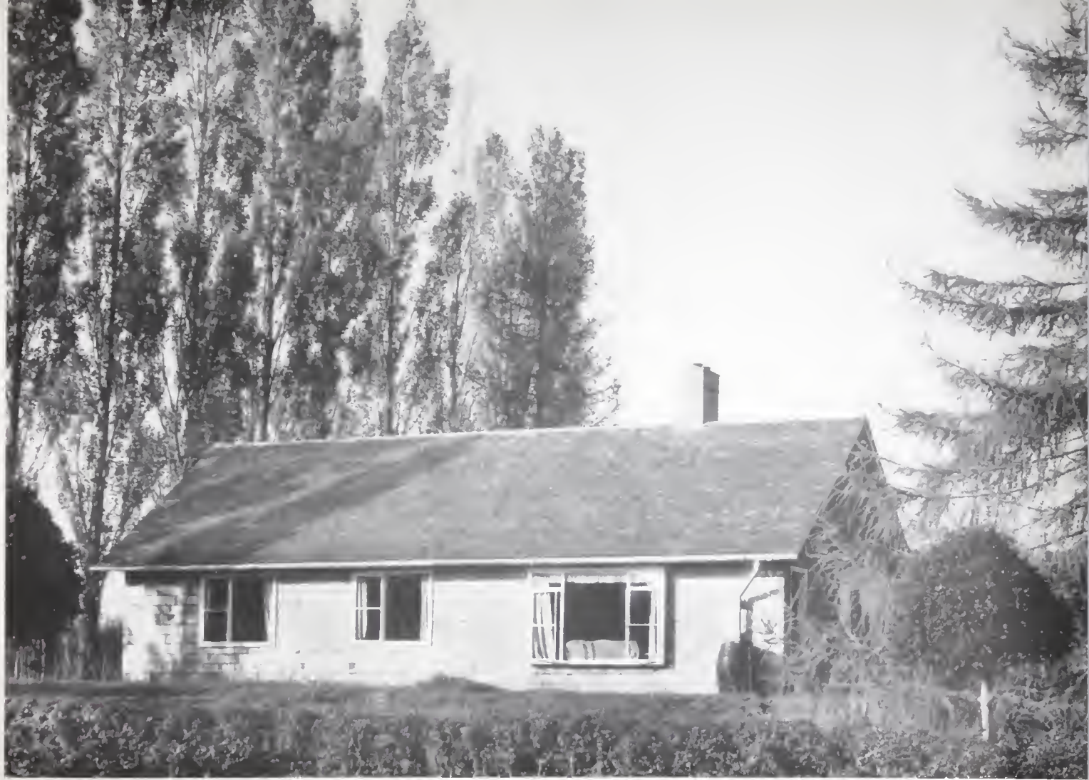
A Colt cottage, Type 9B, with modified windows. Near Tunbridge Wells.
