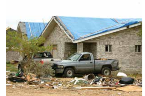
PHOTO: FEMA-provided “blue tarp” temporary roof protection.
