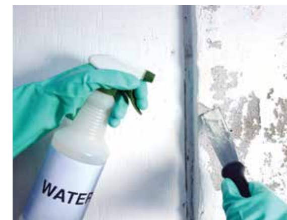
PHOTO: Wet-misting lead paint reduces dust hazard.
