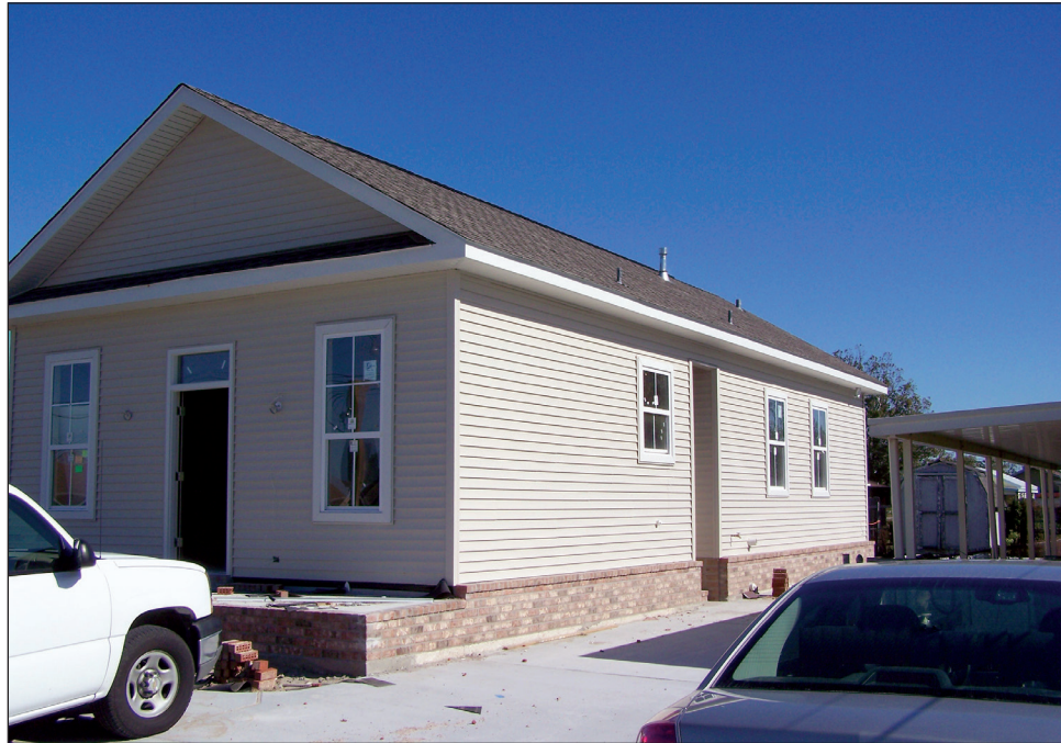
Figure 6-9. Typical mitigation reconstruction project.
