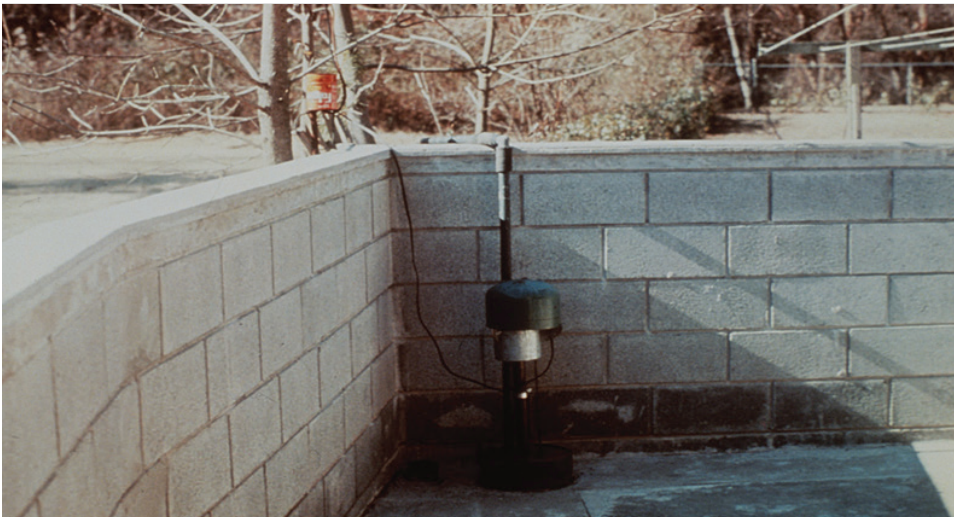
Figure 8-6. Small patio floodwall with sump pump.
