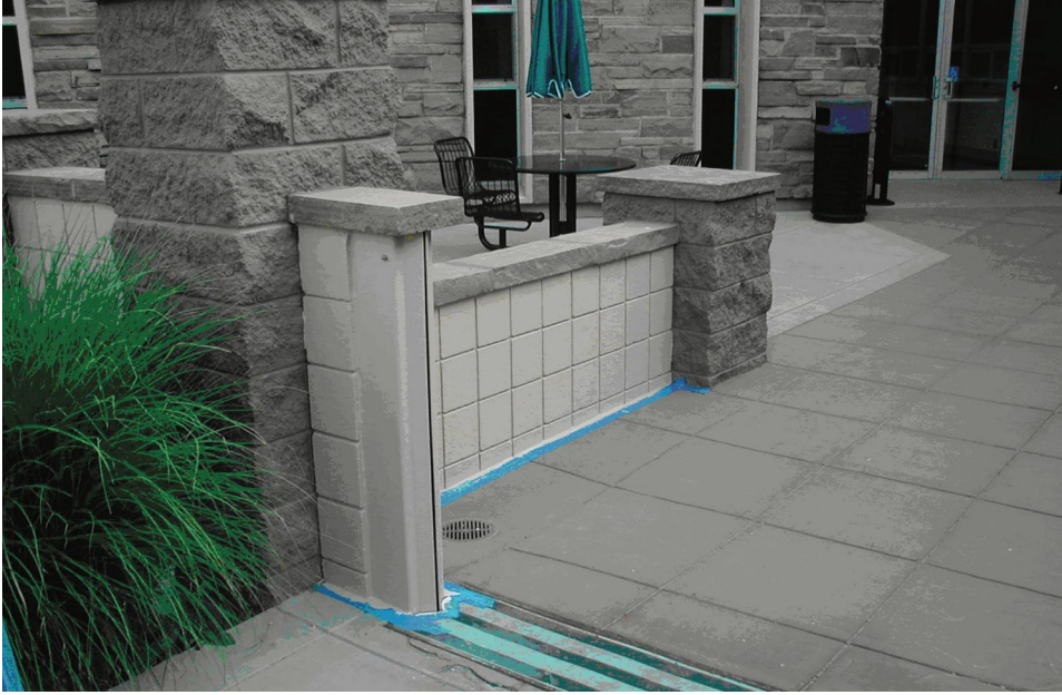
Figure 8-5. The City of Boulder, CO, installed a “pop up” closure to this floodwall at a City office building subject to flash floods. The closure floats up into place automatically when the site is flooded.
