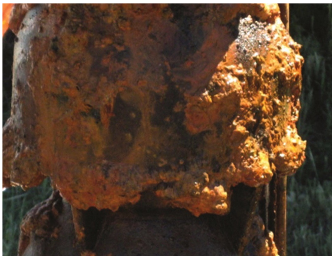
A submersible pump being pulled from a well exhibiting iron oxide, iron bacteria and biofilm.
