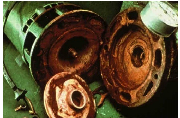
Abrasion caused by pumping sand.
