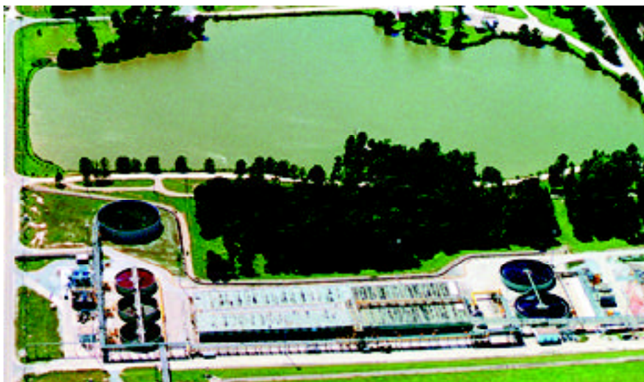
Above ground treatment units at Ciba Specialty Chemicals, McIntosh, Alabama.
