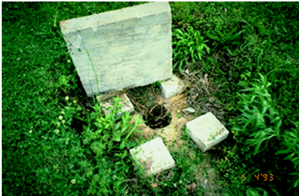
A Class V storm water drainage well in Colbert County. Only a few of these types of wells are known to be in use in Alabama.
