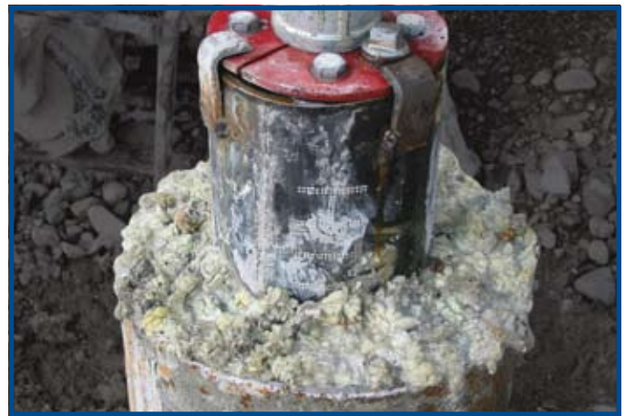
Figure 7. Bentonite cement grout seal between casings.
