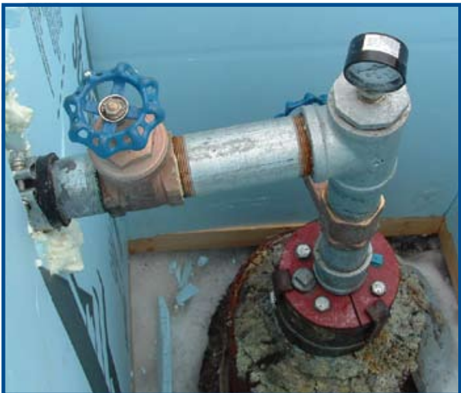
Figure 9. Completed high pressure flowing artesian well.
