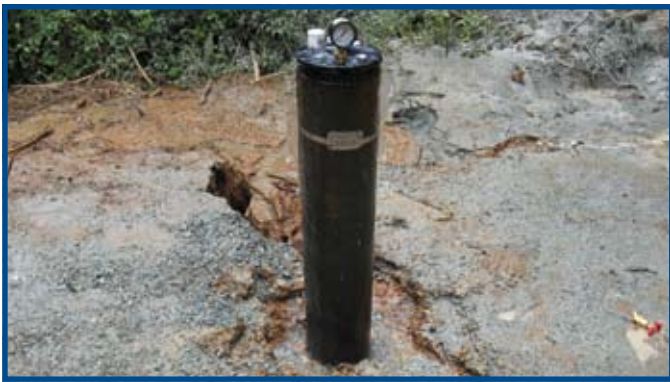
Figure 3. Erosion caused by flowing artesian well.
