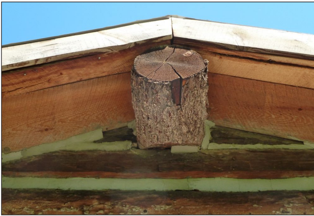
Figure 8. Leaving bark on cabin logs increases likelihood of insect attack and slows drying.
