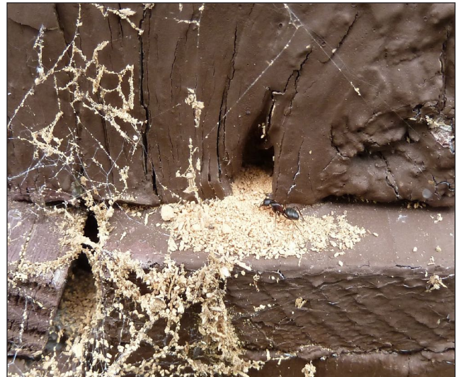
Figure 5. Carpenter ants often reveal their presence with piles of sawdust and frass.
