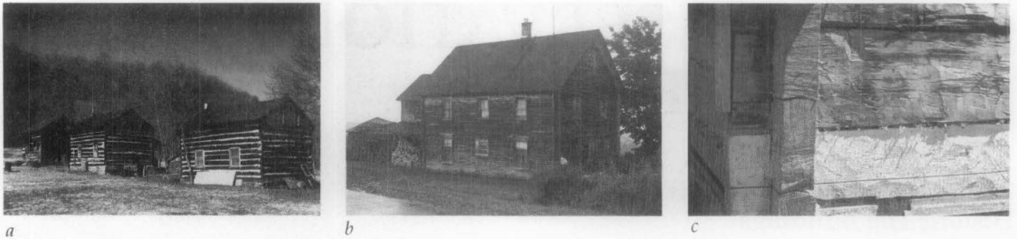
Fig. 2. Logs, both round and hewn, continued to be a basic construction material throughout much of the 19th century, here illustrated by (a) these c. 1831 industrial workers' houses for forgers at the Mt. Etna Iron Furnace in Pennsylvania, and (b) the Larsson-Ostlund House built by Swedish immigrants in New Sweden, Maine, during the 1870s. (c) Corner detail of the Larsson-Ostlund House with the original clapboarding removed during restoration shows close-fitting log joints in the Scandinavian style that did not require chinking. Photos: (a) Jet Lowe, HAER Collection, (b-c) Maine Historic Preservation Commission.
