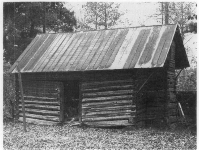
Fig. 15. The mid-19th century O'Quinn House, Moore County, North Carolina, provides a rare surviving example of a clay-lined log chimney. Although the logs of the house are saddle-notched, the chimney logs are "V" notched. The roof was extended out over the chimney to protect the daubing from the weather, and the chimney stack would have originally projected through a hole in the roof. Photo: Michael Southern.
