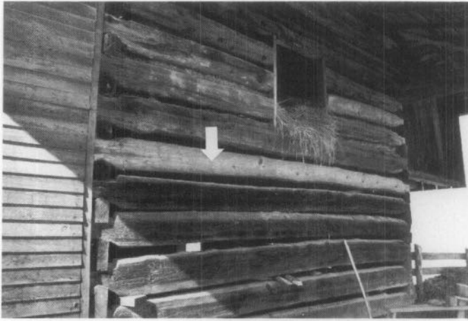
Fig. 22. The lighter-colored replacement log in this barn matches the dimensions and hewing marks of the original logs, and will darken in time to blend visually with the other logs. Photo: Bernard Weisgerber.
