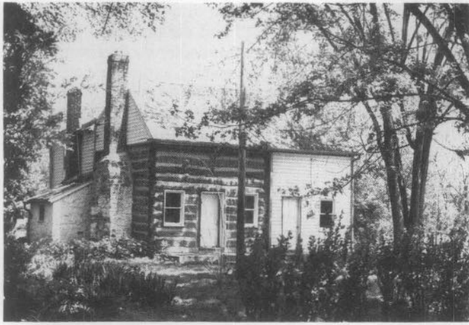
Fig. 13. Historic wood clapboard siding originally applied to conceal the fact that this house was built in two sections of different materials has been inappropriately removed from the 1793 log portion. Photo: National Park Service Files.
