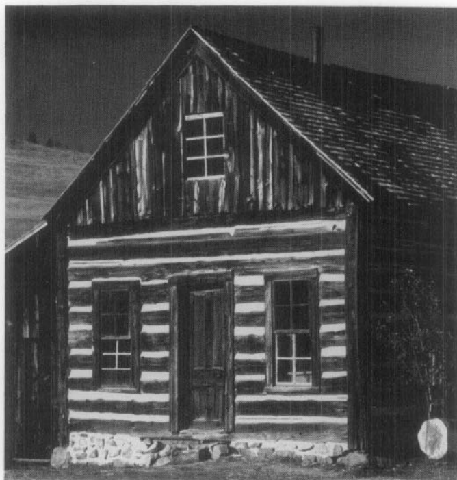
Fig. 9. This historic log building on the Walker Ranch in Boulder, Colorado is an example of the Rocky Mountain cabin form which is typified by the entrance door being located in the gable end. Photo: Bernard Weisgerber.
