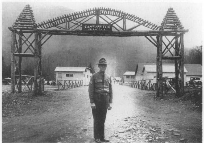
Fig. 7. The Civilian Conservation Corps built many recreational log structures across the country in the 1930s and 40s, including this rustic log gateway to Camp Morton, Lycoming County, Pennsylvania. Photo: Courtesy Lycoming County Historical Society and Museum.
