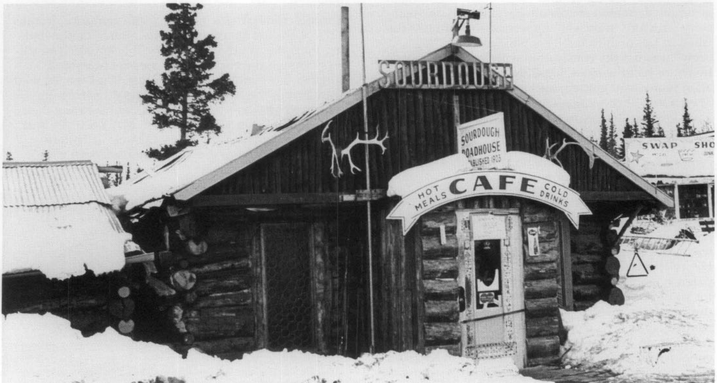
Fig. 1. Log construction was practical in the rough frontier and climate of Alaska, where it was used for a variety of structures such as the Sourdough Lodge (c. 1903) near Gakona. Built to serve the trail leading to the Klondike gold discoveries, this 1-story, L-shaped roadhouse is primarily of horizontal log construction with vertical logs in the front gable. Photo: National Park Service Files.
