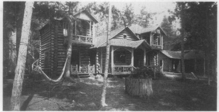
Fig. 5. The main lodge of Echo Camp on Raquette Lake in New York State was built in 1883 by the governor of Connecticut. It typifies the Adirondack style in the use of exposed round logs with crowns, and porches and balconies constructed with banded logs and round log columns. Photo: Courtesy The Adirondack Museum.
