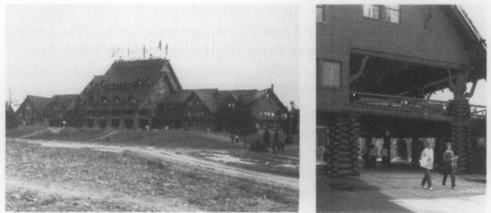
Fig. 6. (a) Old Faithful Inn, Yellowstone National Park, Wyoming, shown here in 1912, brought the Rustic style to the West in 1903 in an original design, and a scale befitting its setting. (b) Although only the first story is of horizontal log construction, the use of logs is striking in the trestle work and cribbed piers around the entrance. Photo: (a) Courtesy National Park Service, (b) Laura Soulliere Harrison.
