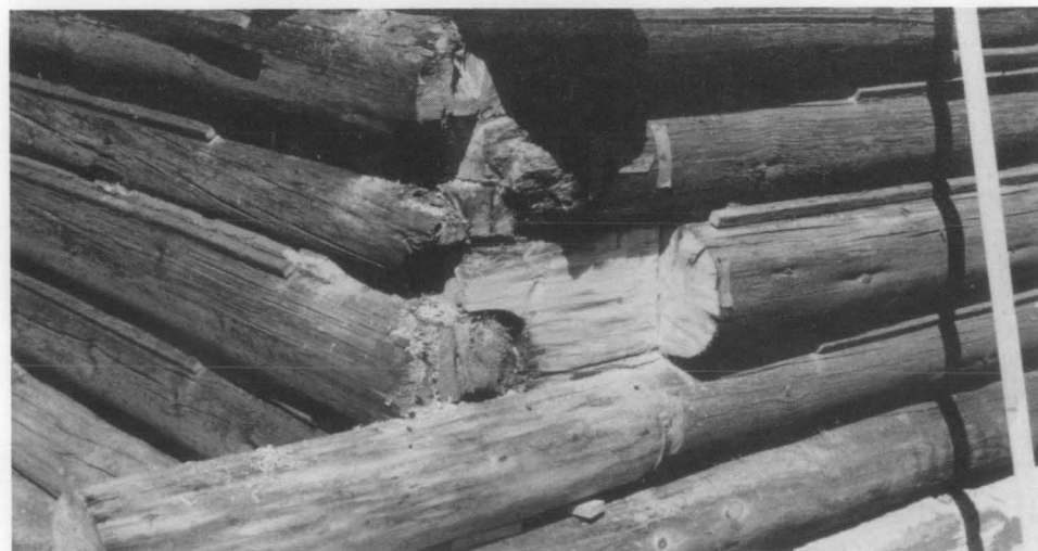
Figure 4. In a few cases, the deterioration had penetrated beyond the center line of the log corners and portions of the wall face were removed. Photo: Harrison Goodall.
