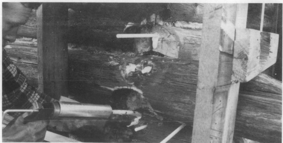
Figure 6. A flexible tube was stapled onto a caulking gun in order to fill the 12"-12 1/2" deep holes that had been drilled into the sound end of the historic log. The individual hole was filled two-thirds with epoxy adhesive and a 1/2" diameter fiberglass reinforcing rebar was then inserted. Photo: Harrison Goodall.
