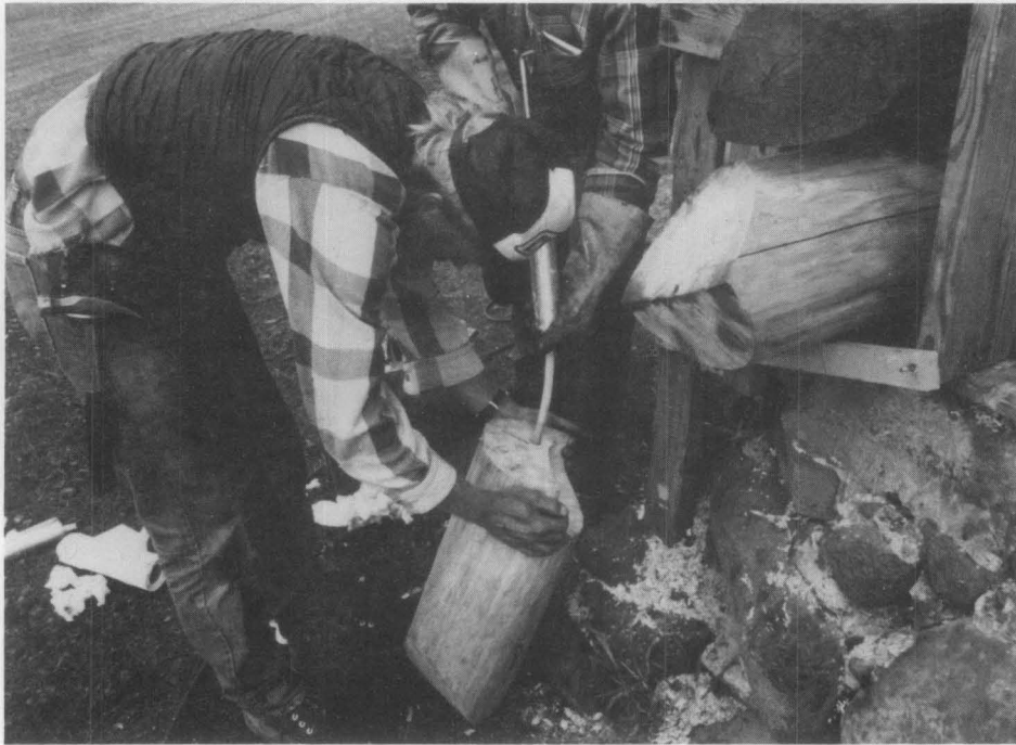
Figure 7. A 12 1/2" long hole was drilled into the new crowns. This hole was filled in the same manner as were the old logs. The crown was then immediately lifted into position and supported by the cribbing framework for several days until the epoxy cured. Photo: Harrison Goodall.
