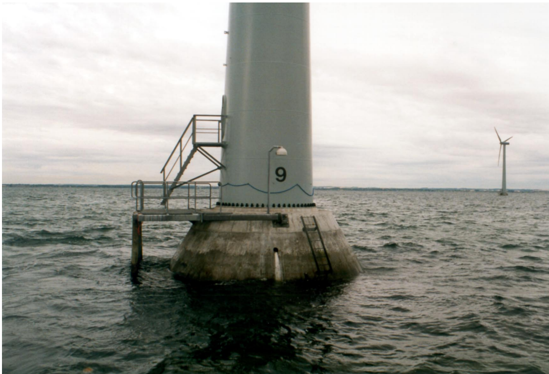
Fig. 2 Offshore wind farm with 0.5 MW wind turbine furnished with ice cones. Tunoe Knob Denmark.
