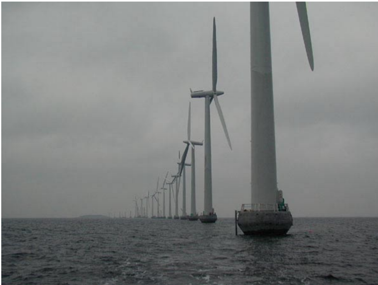
Fig. 3 Offshore wind farm with 2.0 MW wind turbines with inverse ice cones. Middelgrunden, Copenhagen, Denmark.
