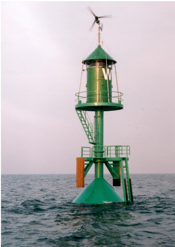
Fig. 1 Light tower W-26 with ice-cone. Access ladder expected to be sheared off in heavy ice.
