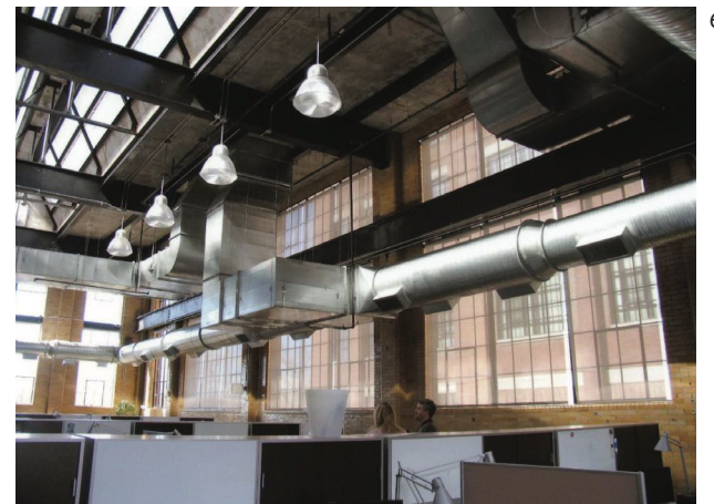
[5-6] Large windows and a roof monitor provide natural illumination in a historic industrial building.
