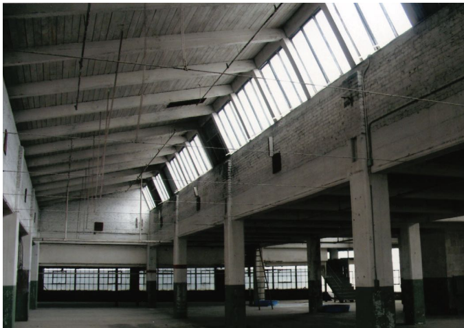
[2-3] Clerestory windows provide natural light in a historic industrial building: Before and after rehabilitation.
