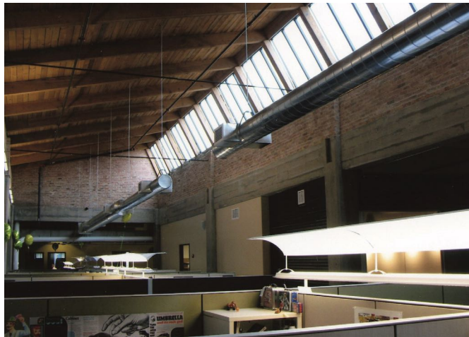
[2-3] Clerestory windows provide natural light in a historic industrial building: Before and after rehabilitation.
