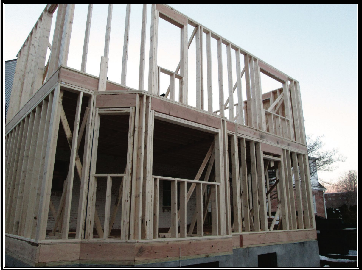
Modern Platform-Framed House Under Construction
