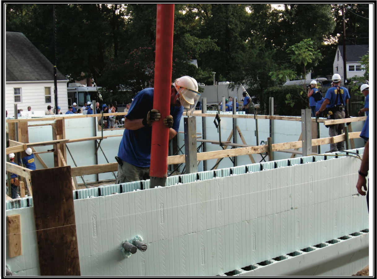
House Construction Using Insulating Concrete Forms
