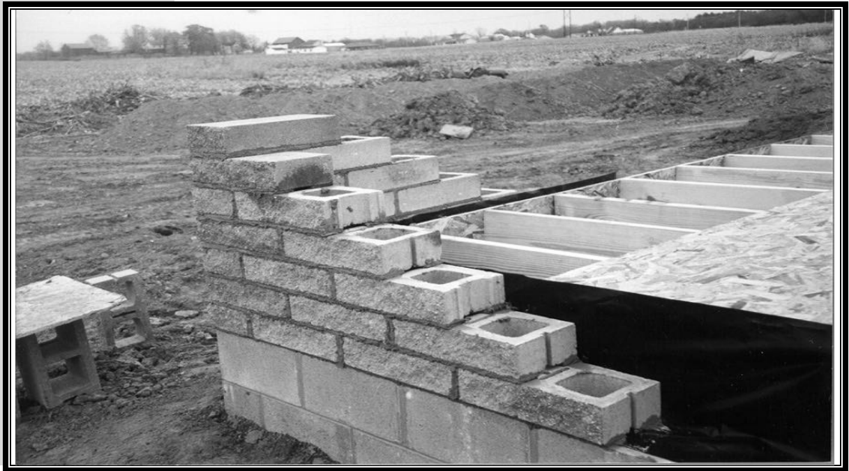
FIGURE 1.6 House Construction Using Concrete Masonry
