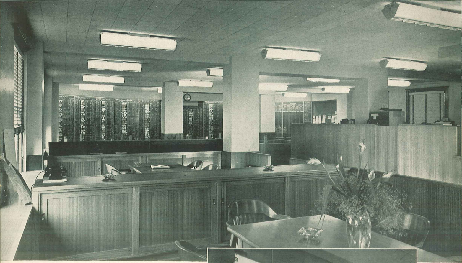
This Fir-Tex Acoustical ceiling treatment gives privacy to each conference within these quarters and adds dignity to the whole.
