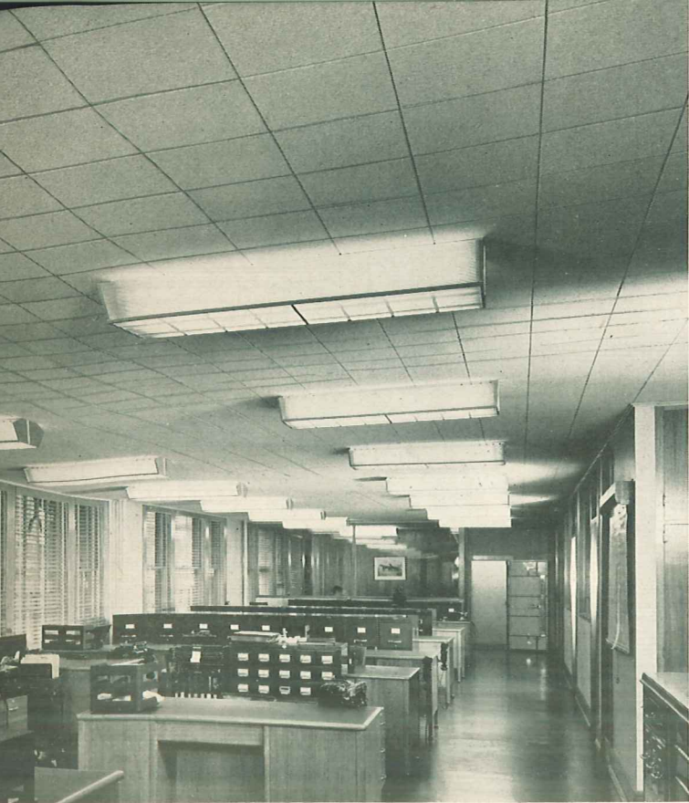
The Fir-Tex Acoustical Tile on the ceiling permits an open arrangement of individual offices within a large room area and maintains privacy in each unit.
