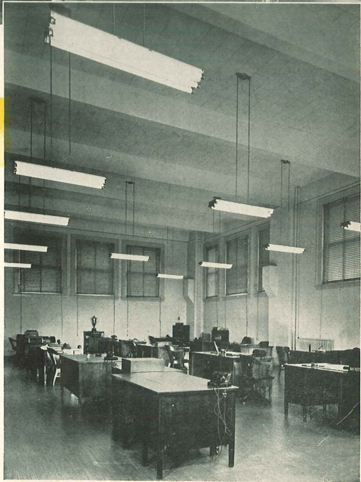
Before this Chamber of Commerce membership room was treated with Fir-Tex Acoustical Tile, there was a bedlam of noise. Now all telephones can be in use simultaneously without anyone disturbing his fellow worker.
