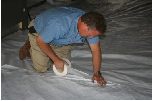
Sealing Floor Liner
