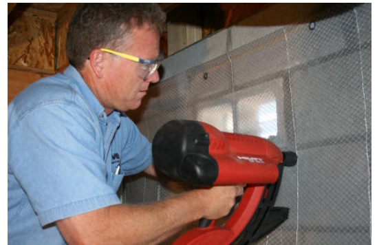
Affixing Wall Liner
