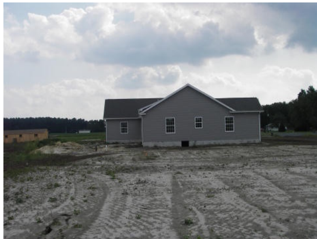
Example of Participating House – Front View
