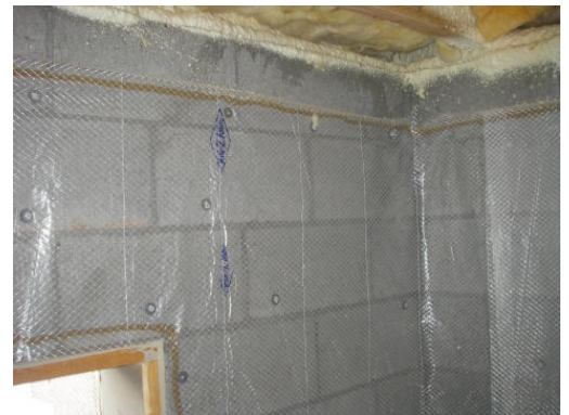
Liner Sealed to Block Wall
