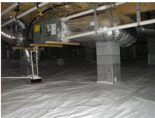
Complete Floor Liner and Wrapped Piers
