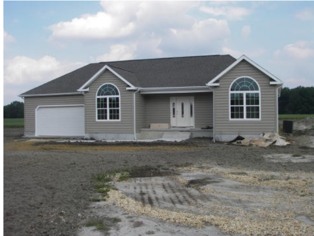
Example of Participating House – Front View
