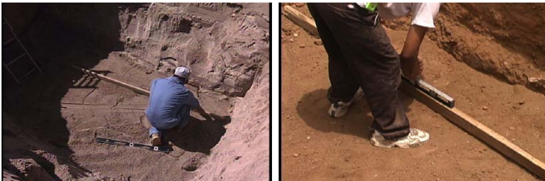
Figure 4. Leveling the bottom of the tank hole.
