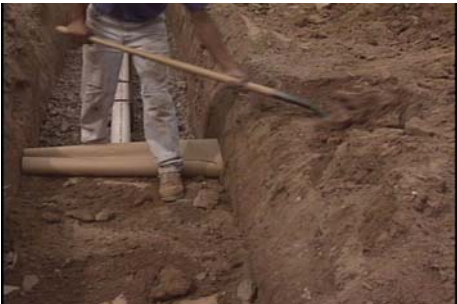
Figure 15. Backfilling the gravel and pipe system.
