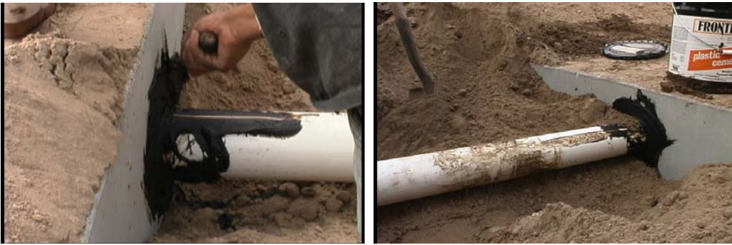
Figure 8. Pipe inlet/outlet joint showing seal
