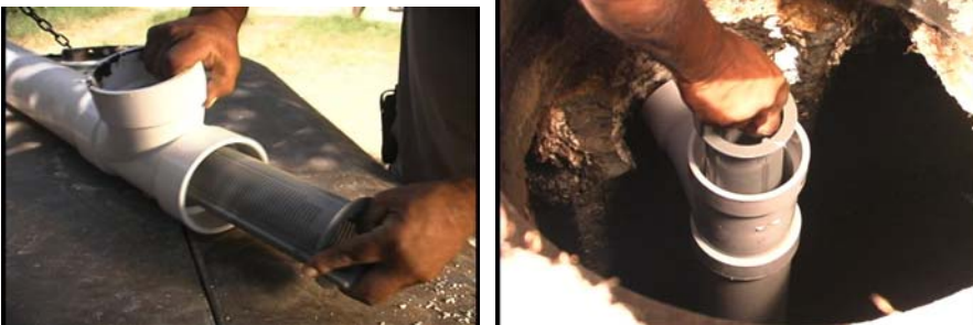
Figure 6. An outlet filter or bioscreen in the septic tank is required.
