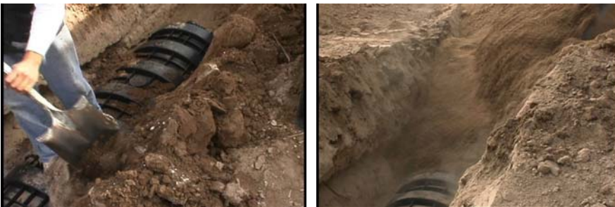
Figure 18. Once the chambers are placed backfill the sides of the chamber prior to backfilling the trench. Failure to do this may result in the chambers collapsing.
