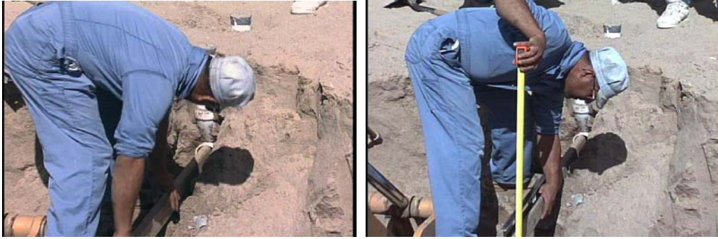
Figure 3. Setting pipe slope using 2x4 and carpenters level.
