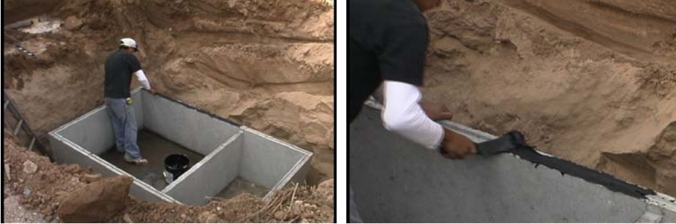
Figure 5. You should be present when your septic tank is installed. If the tank is a split tank make sure the entire joint is filled with mastic prior to tank assembly.
