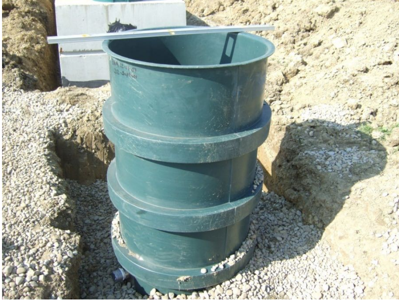
Figure 5. Dosing siphon - external view
