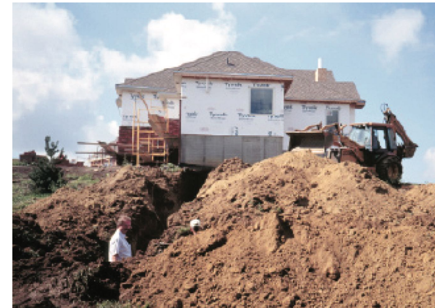
Soils are often disturbed during construction.
