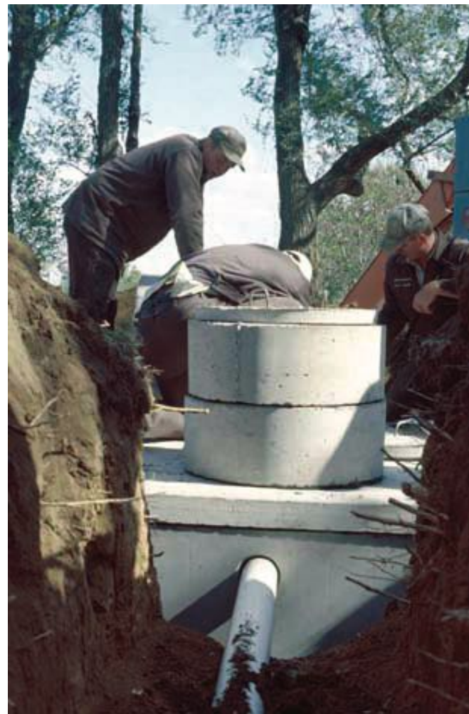
Workers install a new septic system.
