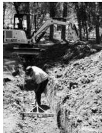
2. Smooth irregularities in the excavation and trench bottom and clear any large rocks or debris from the bottom of the trench. Scarify the soil if smearing is present. Arc by Infiltrator recommends all drainfield trench bottoms or absorption beds should be prepared level. Any allowed slope or fall should be determined and based on your state or local codes.
