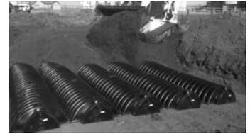
2. Smooth irregularities in the excavation and clear any large rocks or debris from the bottom of the bed. Slope of the bed shall be determined based on state or local code.
