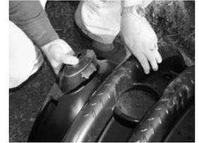
3e. All Arc chambers are designed with an articulating joint that allows for a free-range horizontal rotation of 20 degrees, with a maximum of 10 degrees in either direction. Do not over-rotate the joint beyond 10 degrees. Each Arc chamber is equipped with the “lock & drop” joint which will allow up to 10 degrees of rotation per five foot chamber section.
