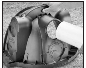
5. Insert inlet pipe.
