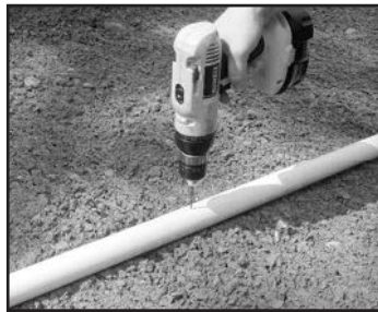
1. Drill hole in pipe.
