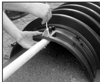
5. Secure pipe to chamber.
