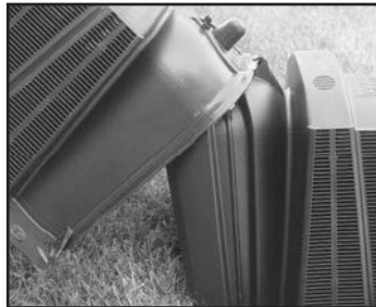
8. Attach endcap to chamber.
