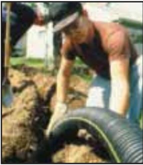
According to the EPA, the gravel in a conventional pipe and gravel system performs three basic functions: 1) its void spaces provide storage capacity for the effluent; 2) it protects the infiltrative surface area of the soil; 3) it supports the excavation. The gravel does not digest, treat or eliminate the effluent.
