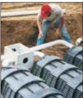
Gravel-less systems include SB2® pipe, Multi-pipe systems, GEO-flow pipe and HDPE leaching chambers. These are the most commonly used conduits in gravel-less systems.
