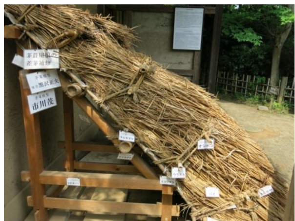
Fig 80. Thatched roof structure model.
