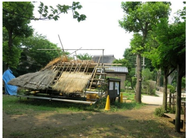
Fig 89. Thatching on a low roof model.
