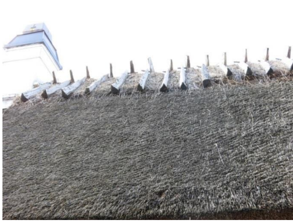
Fig 22. The cut roof surface.
