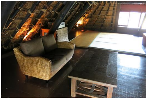
Fig 33. The inn's inner roof.
