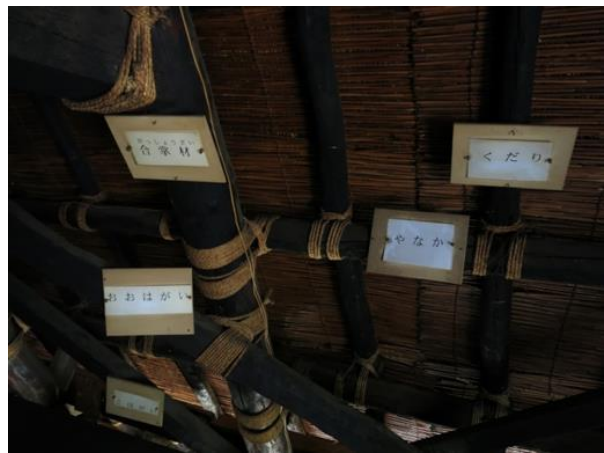
Fig 68. Name tags on the roof structure.
