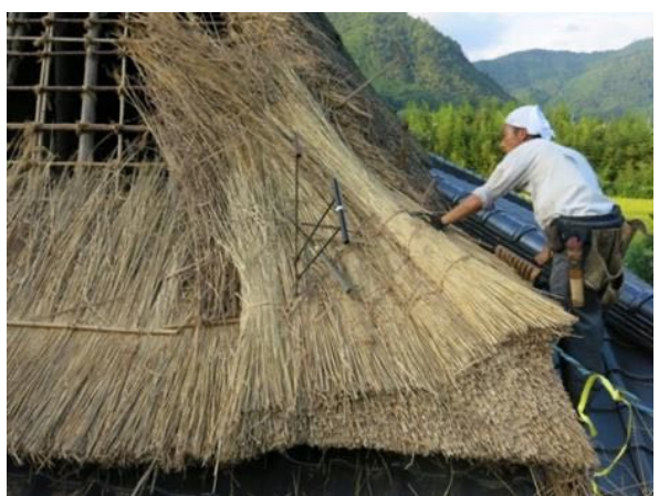
Fig 11. Making the corner and the next layer.
