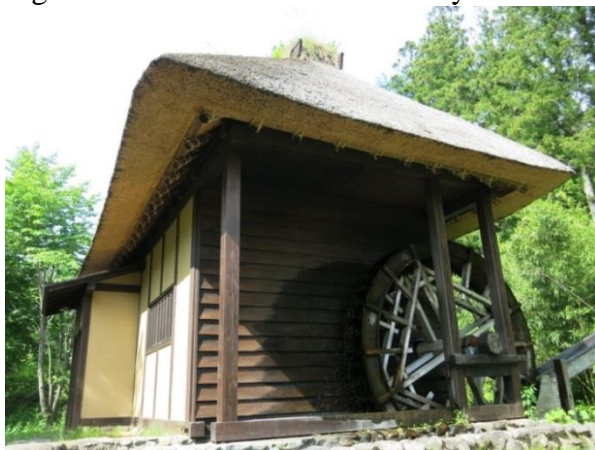
Fig 99. A water mill in use.
