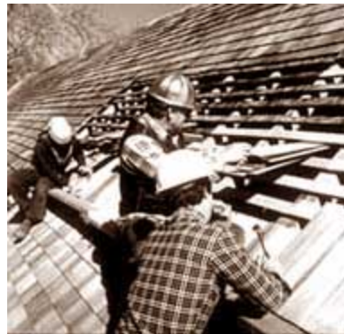
Appropriate re-roofing work in progress. Photo: NPS files.
