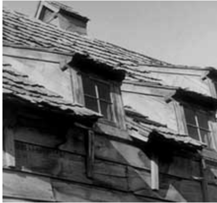
The long, biaxially tapered handsplit shingles are overlapped both vertically and horizontally. Photo: NPS files.
