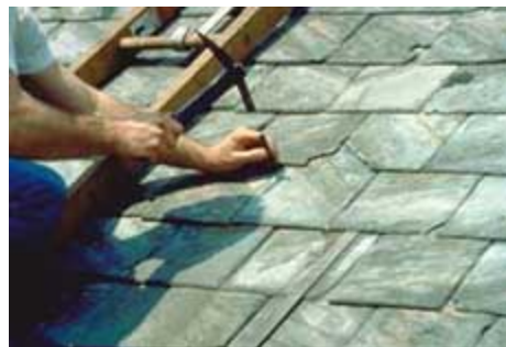
Slate roof repair. Photo: Jeffrey S. Levine.
