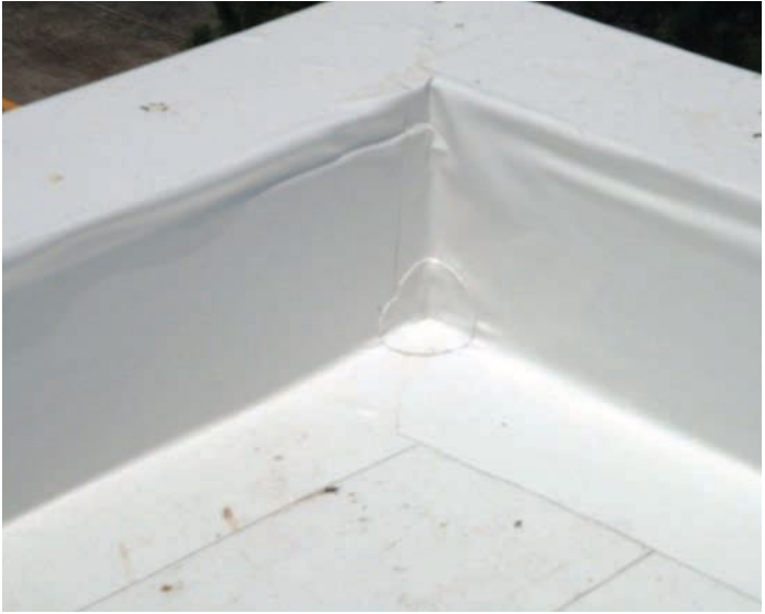
Pre-formed inside corner flashing
