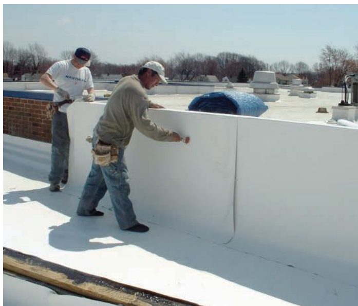
Rolling wall flashing into place
