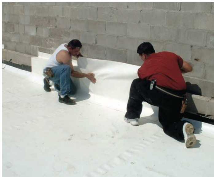
Hanging the wall flashing
