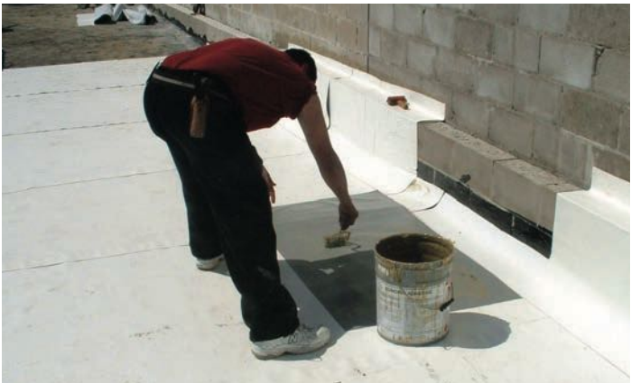
Applying flashing adhesive
