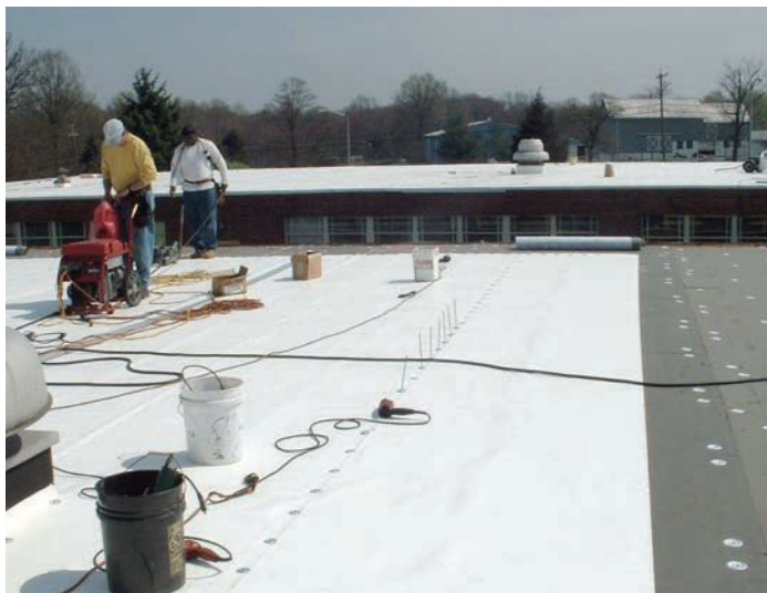
Mechanically fastened Flex TPO membrane
