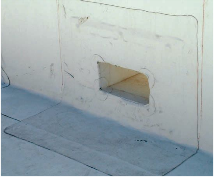
Through-wall scupper made of FlexClad™ Metal
