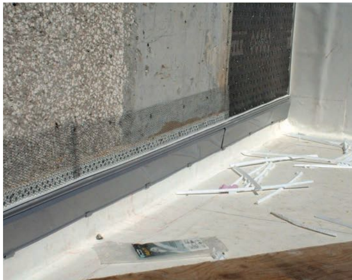
Wall flashing with metal counter-flashing
