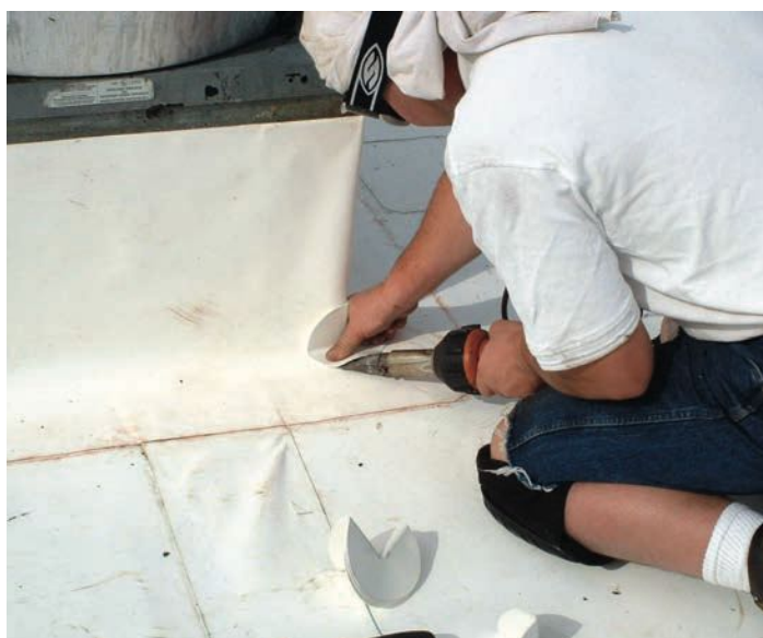
Hand welding a pre-formed outside corner flashing
