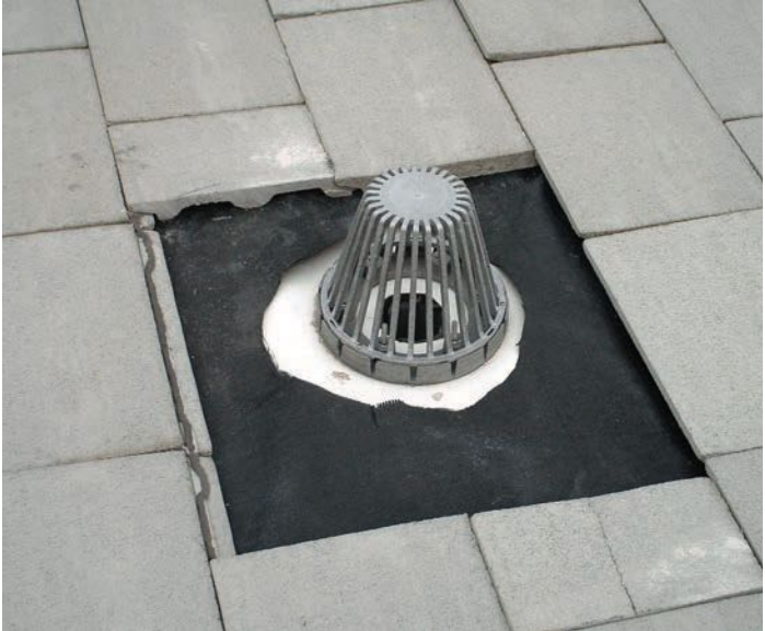
Pavers installed over properly flashed drain detail
