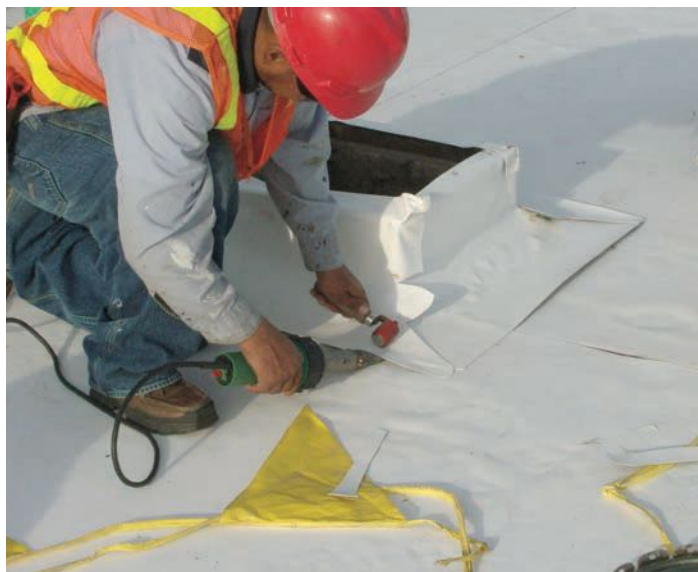
Hand welding a field-fabricated flashing
