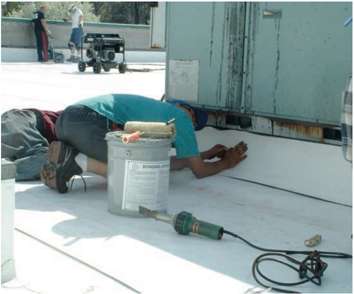
Flashing existing mechanical unit
