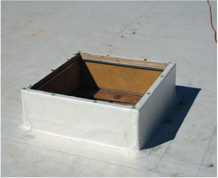
Flashing on an open top curb
