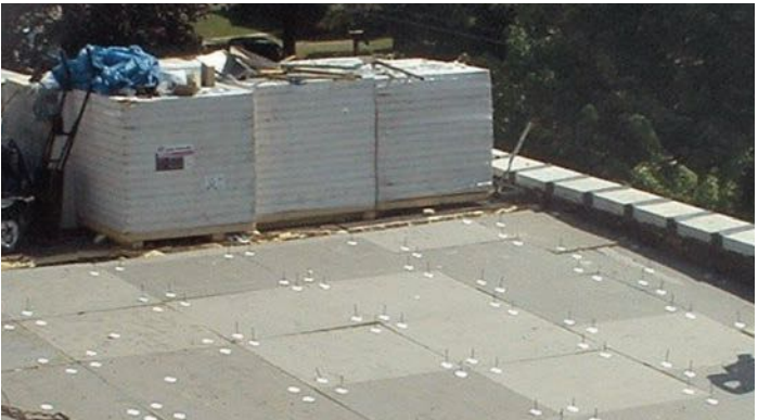
Mechanically fastened Flex insulation board
