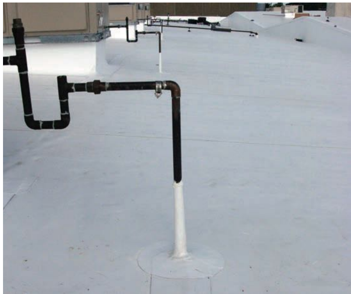
Field-fabricated method with Flex TPO Flashing Membrane
