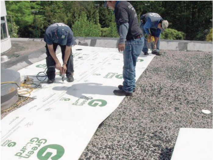
Placing Flex fan-fold GreenGuard re-cover board
