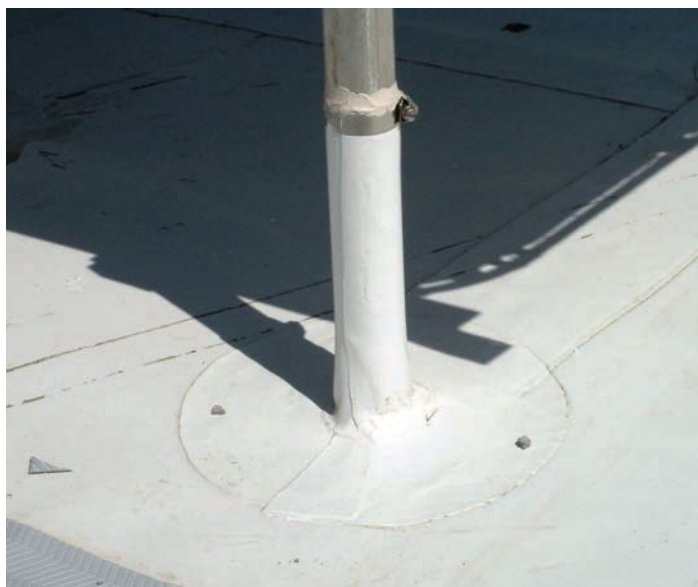
Flex Split Pipe Boot, a pre-fabricated flashing
