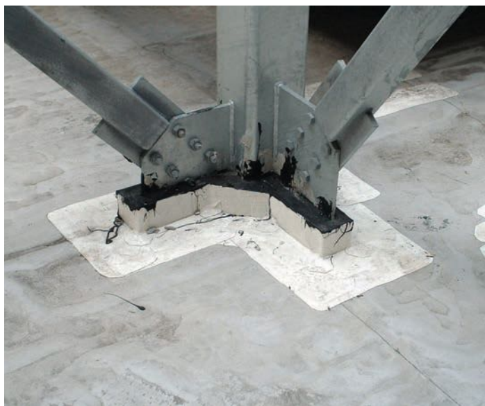
Pitch pans solve difficult flashing details
