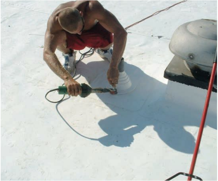
Welding a Flex pre-formed pipe boot to the field membrane
