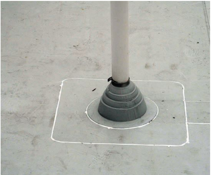
Clamp and caulking is required at the top of the pipe boot
