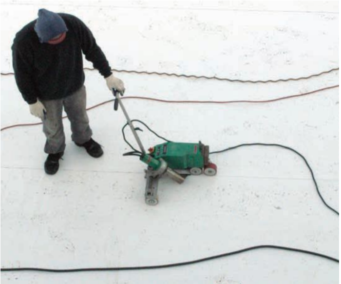
Automatic hot air welder allows workers to operate upright, which is more comfortable and much faster.
