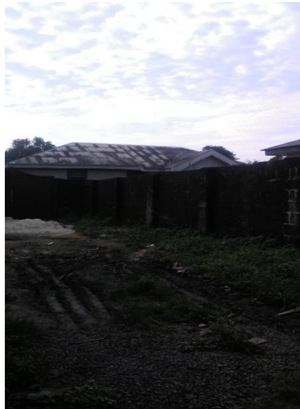
Fig. 2. Building Roof Completely Covered with Dark-Black Coating/Deposit.
