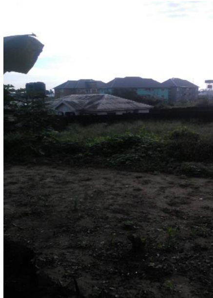
Fig. 4. The Roof Top of the Building in the Front is covered with Dark-Black Deposit, the Storey Buildings Behind are Roofed with Dark-colour Roofing Sheets to Conceal the Effect of the Dark-Black Deposit.
