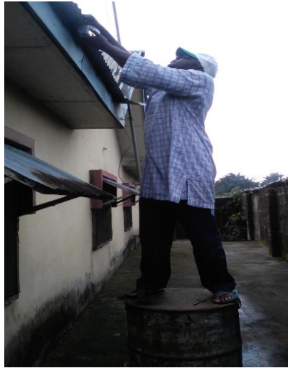
Fig. 7. Field Work and Sample taking in Progress.
