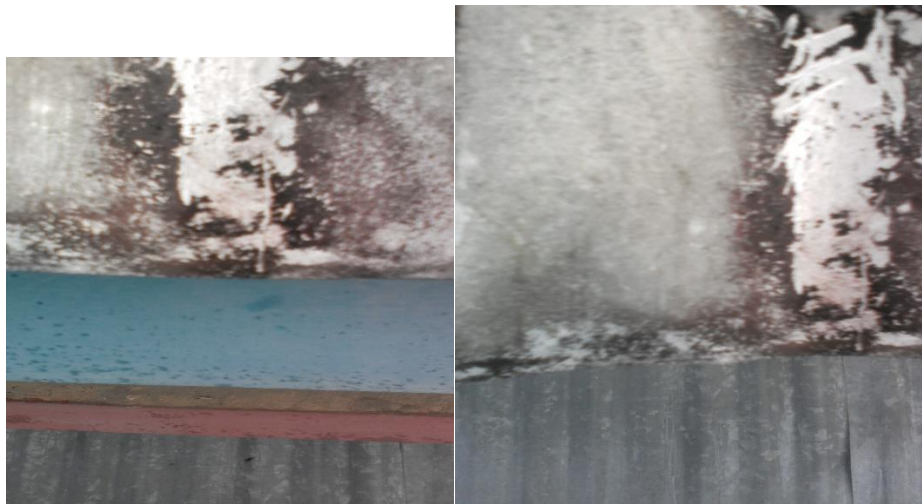
Fig. 8. Roofs showing Reflective Surfaces where test specimens were scrapped from the roofs.
