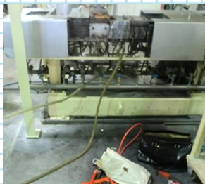
Fine cooling water piping
