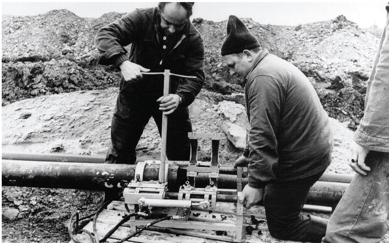
Polybutene piping being installed over 40 years ago
