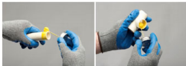
Image 6 and 7. Cement application
