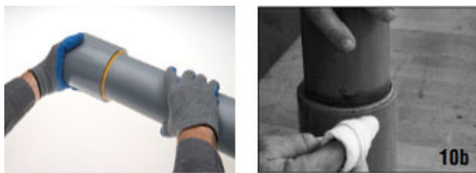
Image 19 and 20. Joining and Cleaning
