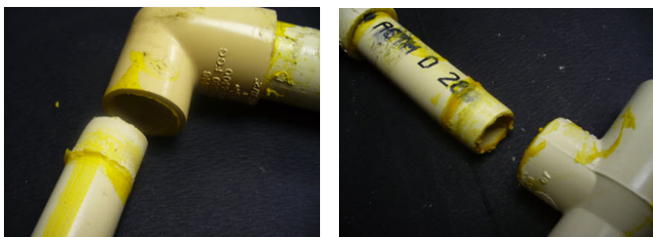
Image 22 and 23. Insufficient cement/dry joint
