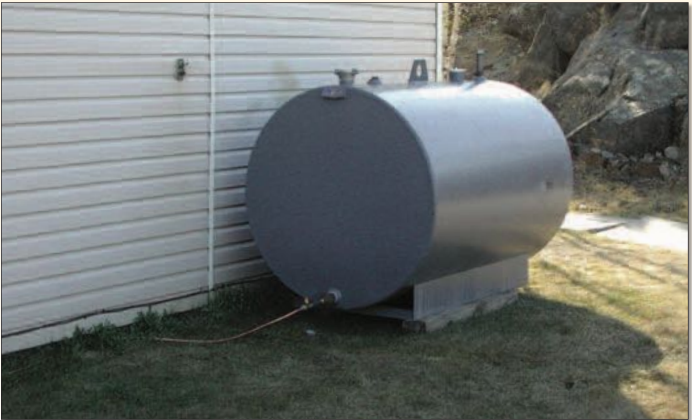
Double-wall steel heating oil tank.
