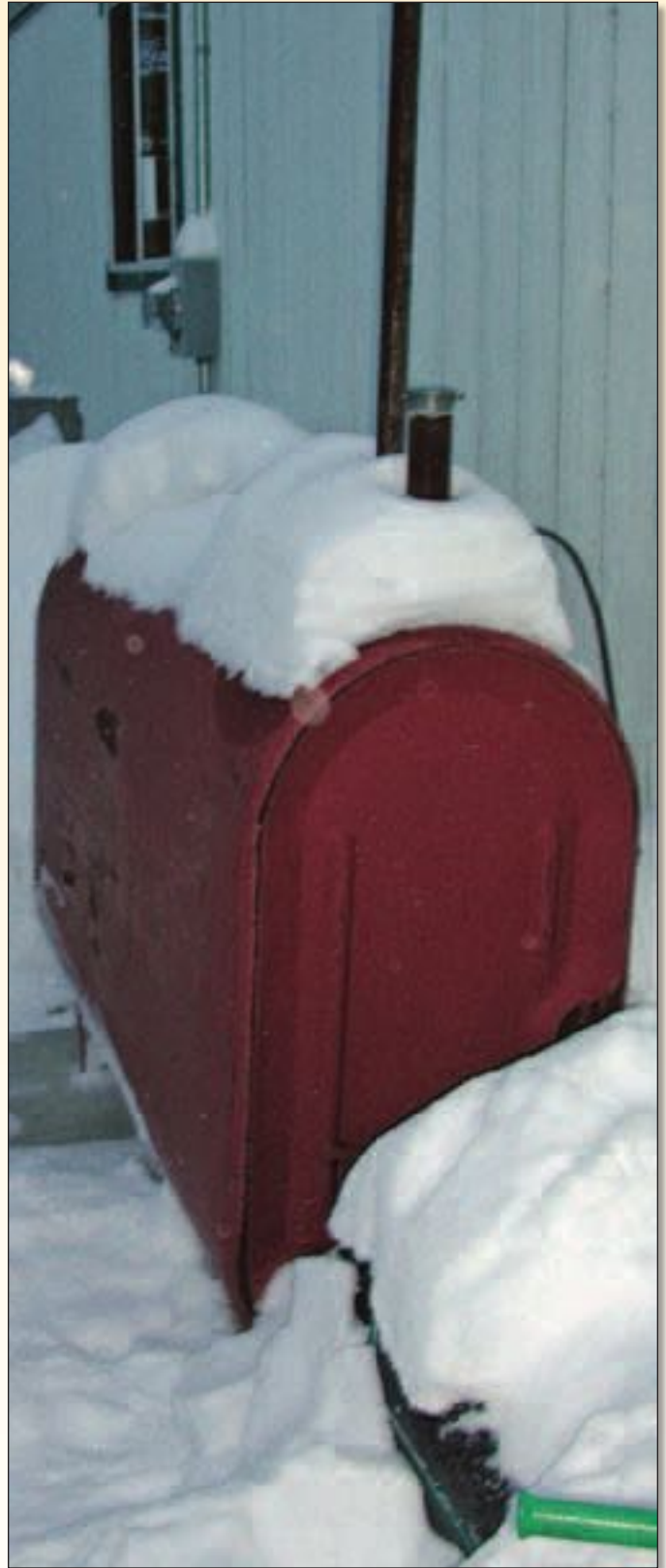
Typical oil tank location.
