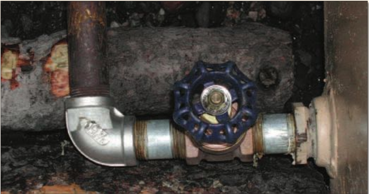
Newly installed oil tank valve. Note the oil stained ground still requiring clean-up.
