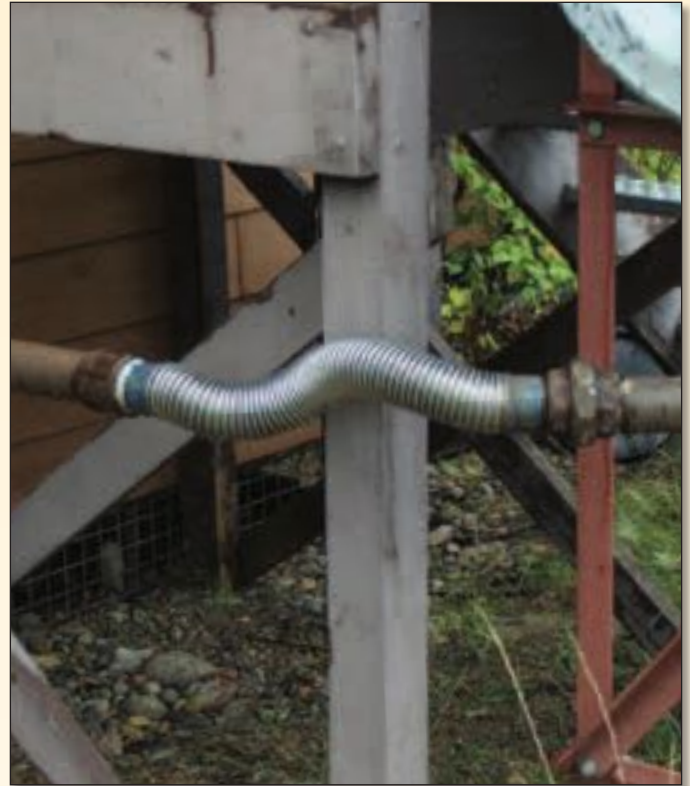
This flex connector is out of alignment.
