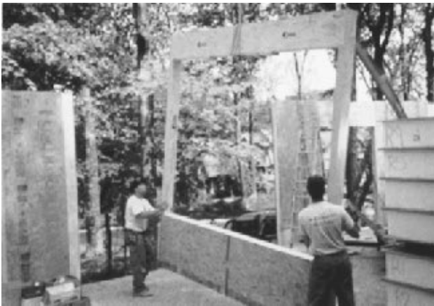
Figure 15.7 SIP installation. ( R-Control Building Systems )
