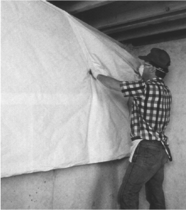
Figure 8.10 Polypropylene-faced fiber glass roll. ( CertainTeed )
