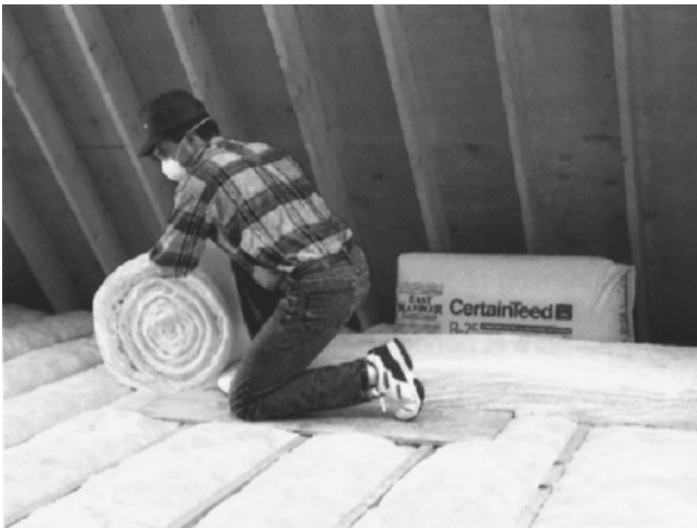
Figure 8.9 Encapsulated fiber glass insulation. ( CertainTeed )
