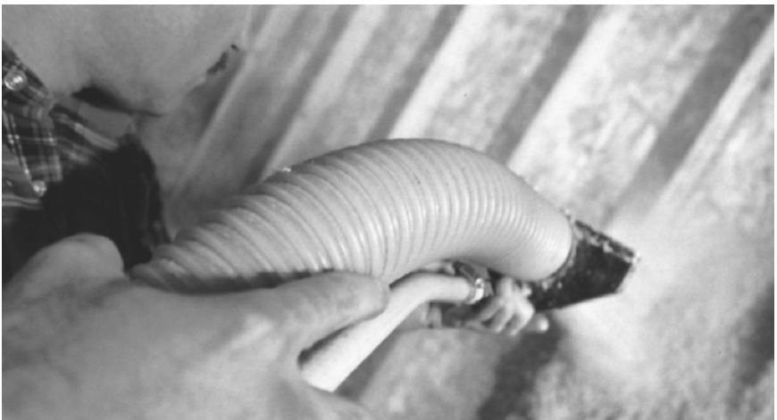
Figure 9.1 Applying wet-spray cellulose. (Greenstone)
