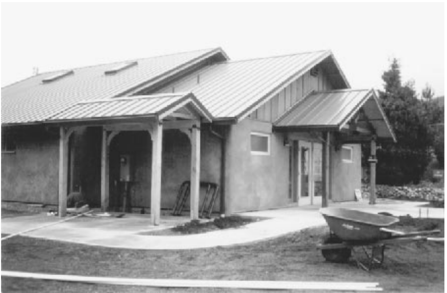
Figure 15.33 Conventional roof. ( Harvest Built Homes )
