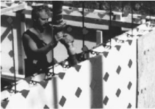
Figure 15.15 Installing ICF. ( R-Control Building Systems )
