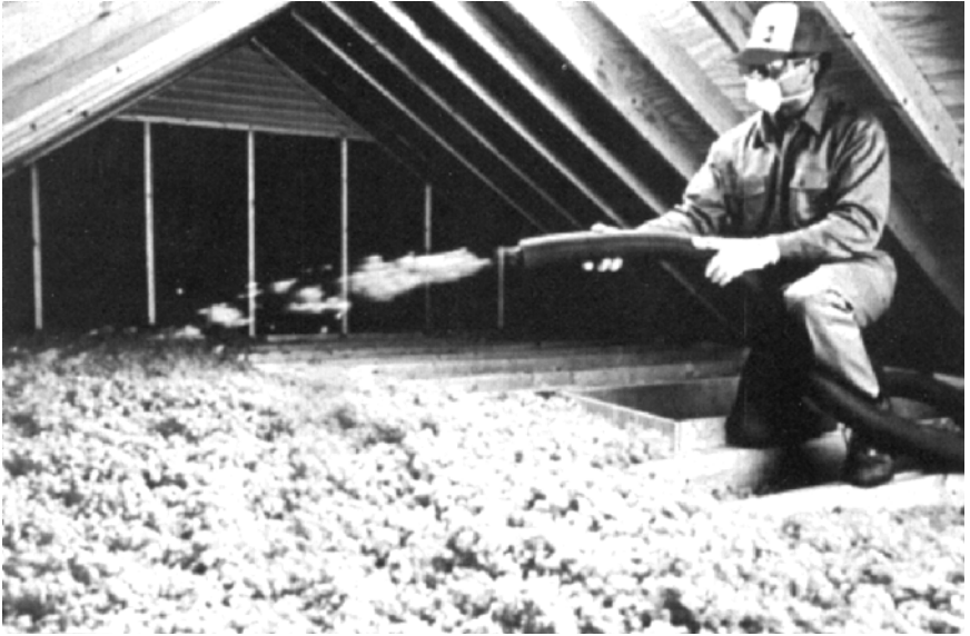
Figure 7.1 Blowing loose fill insulation. (NREL/DOE)
