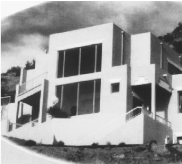
Figure 15.19 Finished construction. ( American Polysteel, Inc. )
