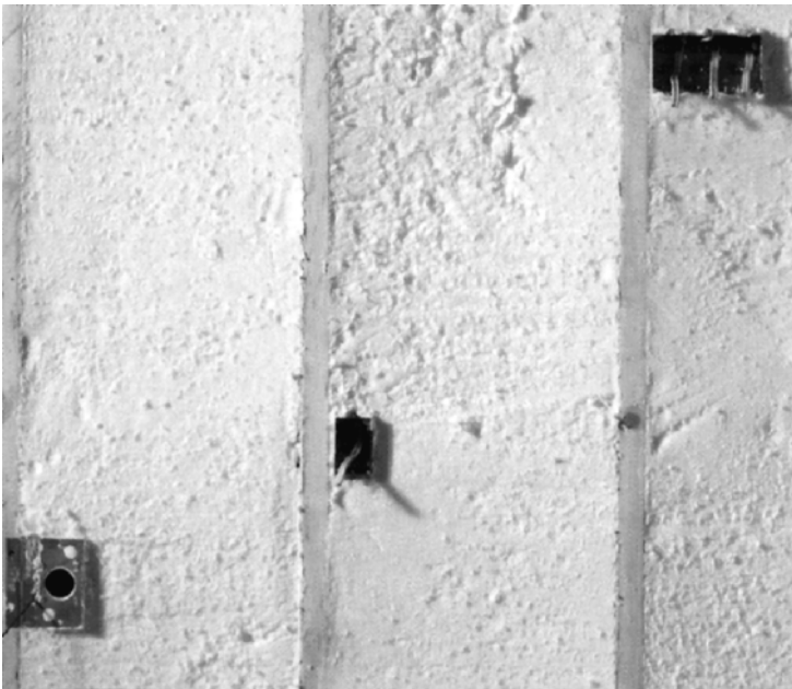
Figure 10.2 Icynene after being scarfed. ( Icynene )
