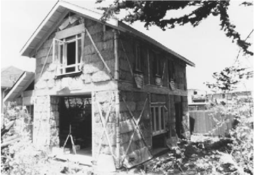
Figure 15.36 Berkeley cottage under construction. ( Daniel Smith & Associates, Architects )
