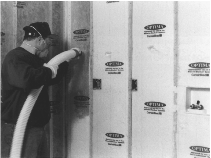
Figure 9.7 Installing the blow-in-blanket system. (CertainTeed)
