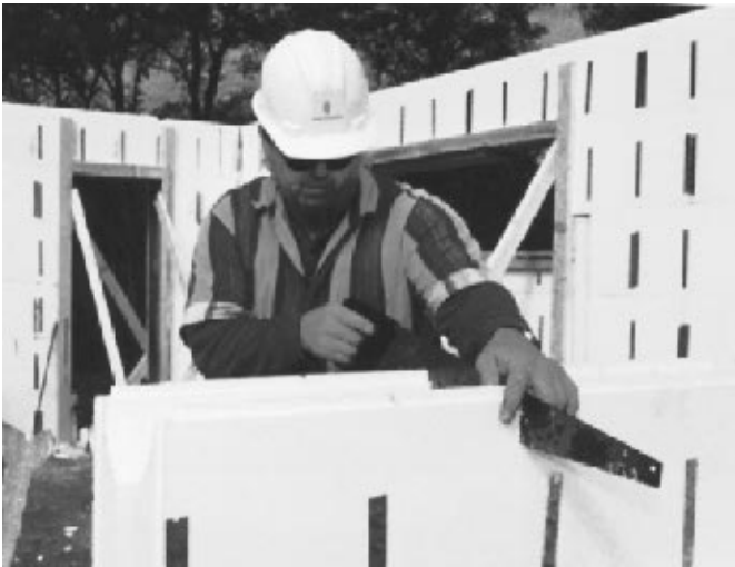
Figure 15.20 ICF Installation. (American Polysteel, Inc.)
