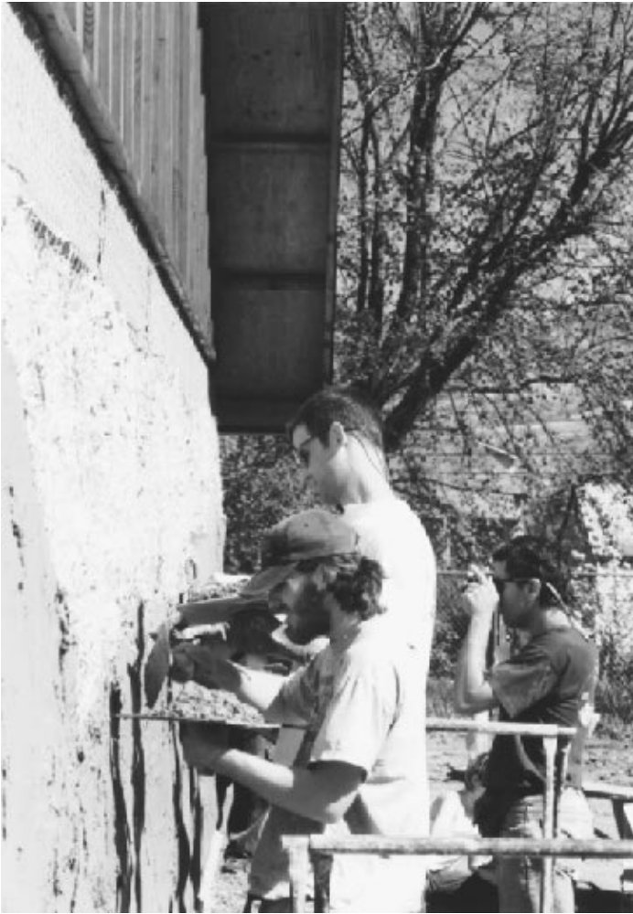
Figure 15.30 Stucco application. ( Harvest Built Homes )
