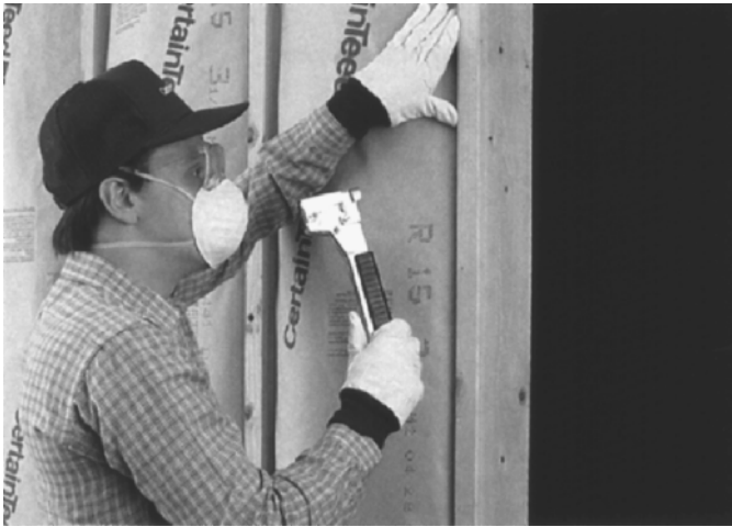
Figure 8.7 Installing batt insulation. ( CertainTeed )
