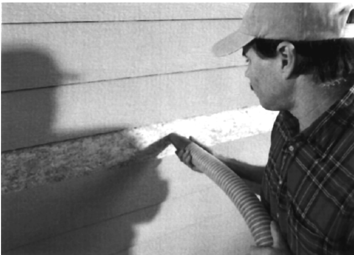
Figure 7.3 Cellulose installation by pneumatic equipment. ( Greenstone )
