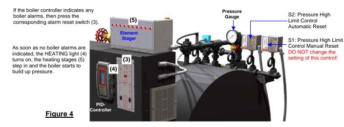
Observe pressure gauge while pressure builds up. The working pressure has been factory set to your specification. As soon as the boiler pressure approaches the pressure setting in the PID-controller, the heating stages of the Element Stager begin to step out. As soon as the boiler pressure reaches the pressure setting in the PID-controller, all heating stages should be off. If you wish to change the working pressure setting, proceed as follows:
