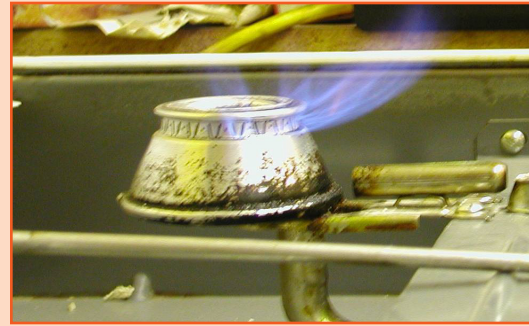
Dirt or rust prevents an even flame on this cook stove burner and causes CO to be produced. The gas openings were cleaned with a pipe cleaner to eliminate CO and allow an even, clean-burning flame.
