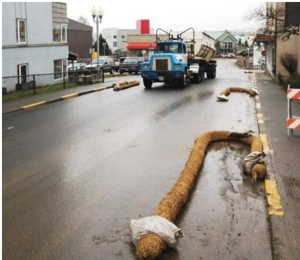
Figure 11. Sawdust-stuffed burlap tubes are weighed down with sandbags in 'U' and 'J' shapes (EPA photo courtesy John Pavitt, Region 10).
