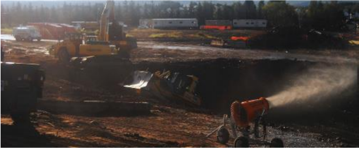
Figure 13. A machine delivering an atomized mist keeps materials adequately wet. This work is being conducted at a lead-remediation site with compliance requirements similar to the Asbestos NESHAP. (Photo used with permission from DustBoss, 2015). No endorsement is implied. Illustration provided for informational purposes only.
