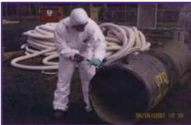
Figure 5.5: Asbestos pipe removalists undertaking removal works
