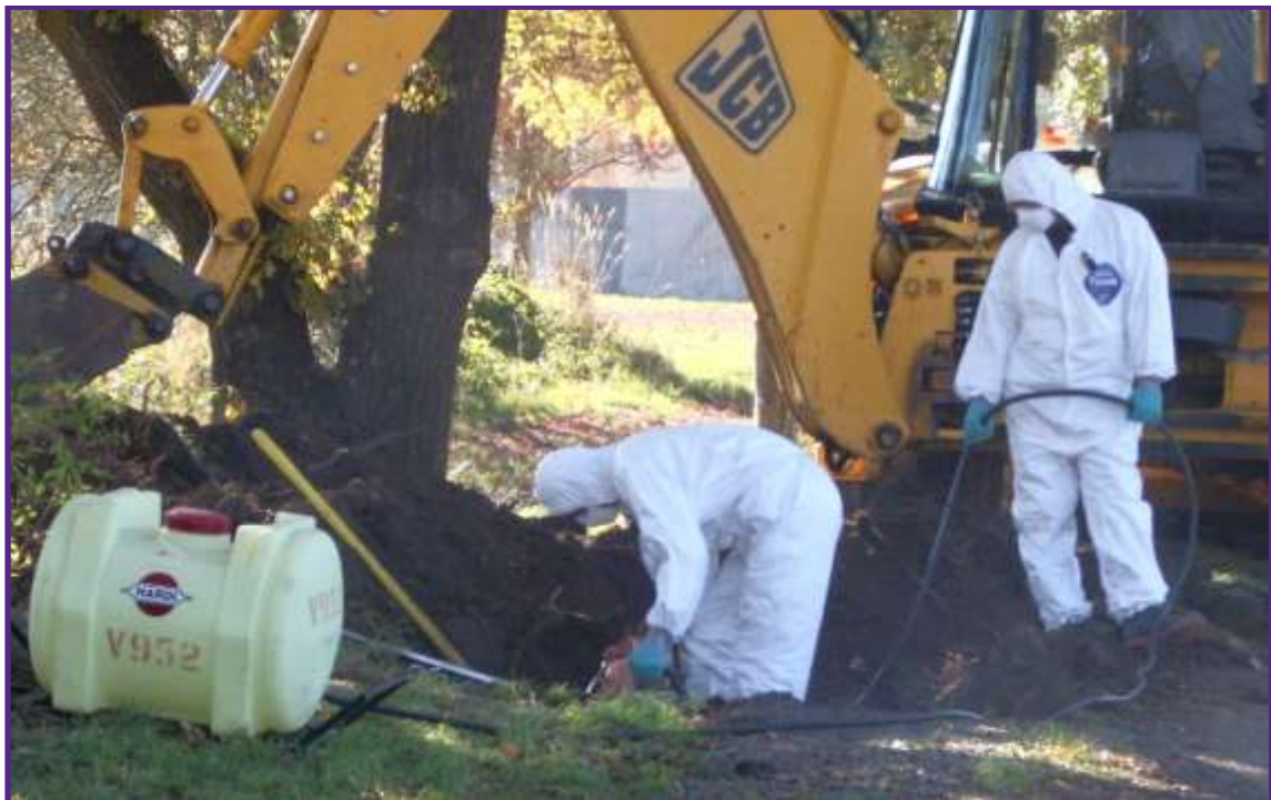
Figure 6.3: AC water main pipe removal using a demolition saw and with water continuously running
