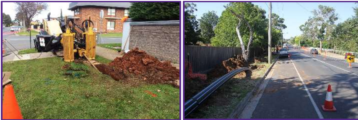
Figure 3.3: SE Water using the realign and leave technique for pipe renewal
