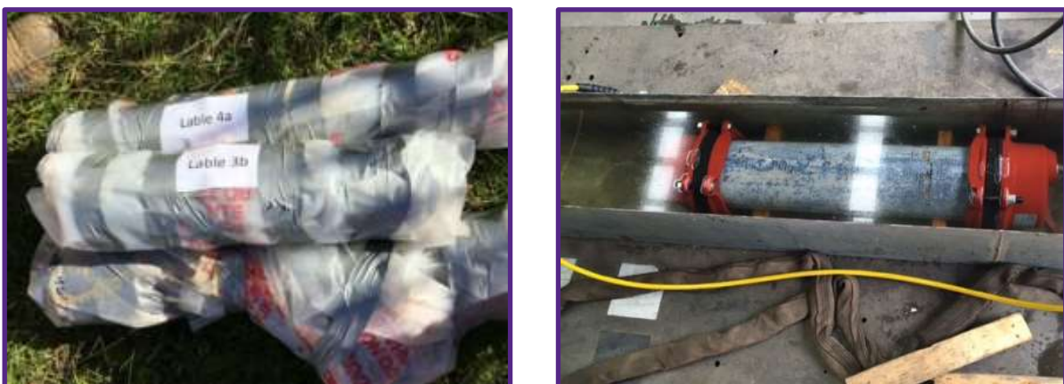
Figure 3.4: Example AC pipe renewal techniques that have been considered (left image is exhumed cured in place samples that were extracted to be laboratory tested, right is cured in place break test apparatus being tested)
