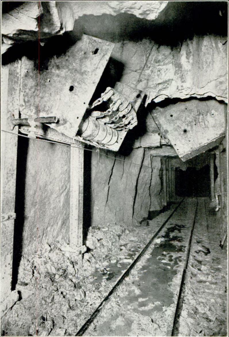
FIGURE 7.—Steel chutes and chain-chute gates, Asbestos Corporation, Ltd., mine, Thetford Mines, Quebec.
