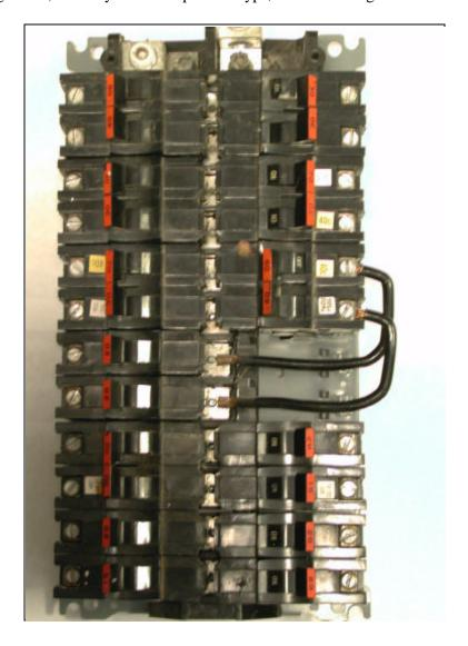
FIGURE 8 - FPE STAB-LOK® "RULE-OF-SIX" (SPLIT-BUS) PANEL WITH NO MAIN BREAKER. THE JUMPER CABLES ON THE RIGHT SIDE FEED THE LOWER SECTION.
