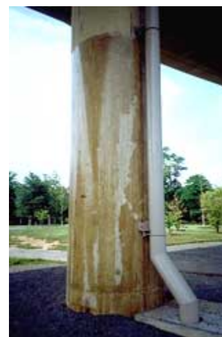
This formerly clear barrier coating is very shiny and has discolored as it has aged. Photo: NPS files.
