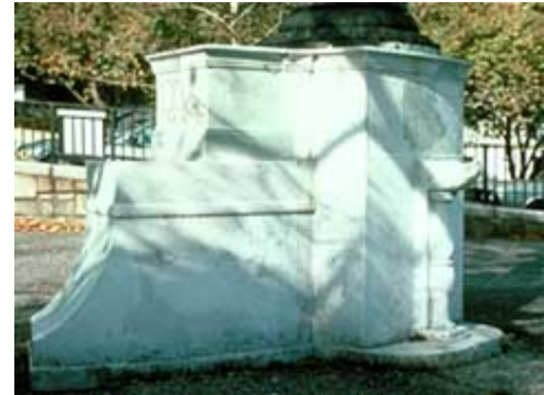
Painting over graffiti on stone is not a recommended maintenance treatment. Photo: NPS files.
