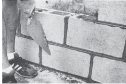
Remove excess mortar burrs
