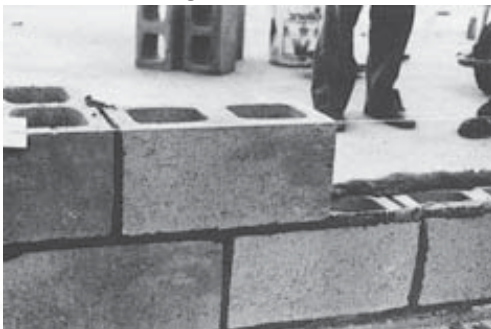
Lay blocks to mason's line
