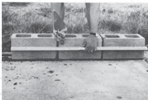
Check alignment with straightedge
