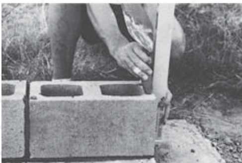
Check corner for plumb
