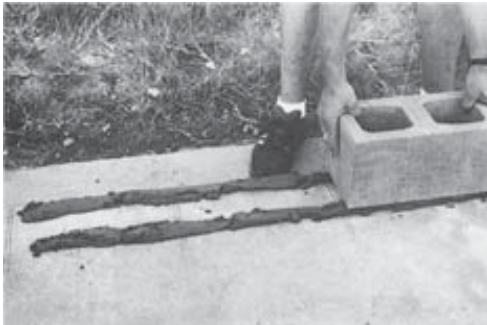
Positioning first corner block
