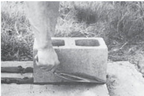
Remove excess mortar
