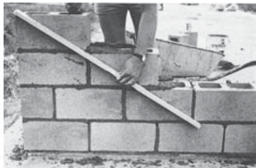
Check corner alignment
