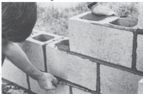
Tool horizontal joints
