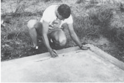
Setting out to block modules
