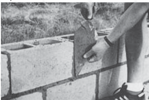
Re-fill mortar joints
